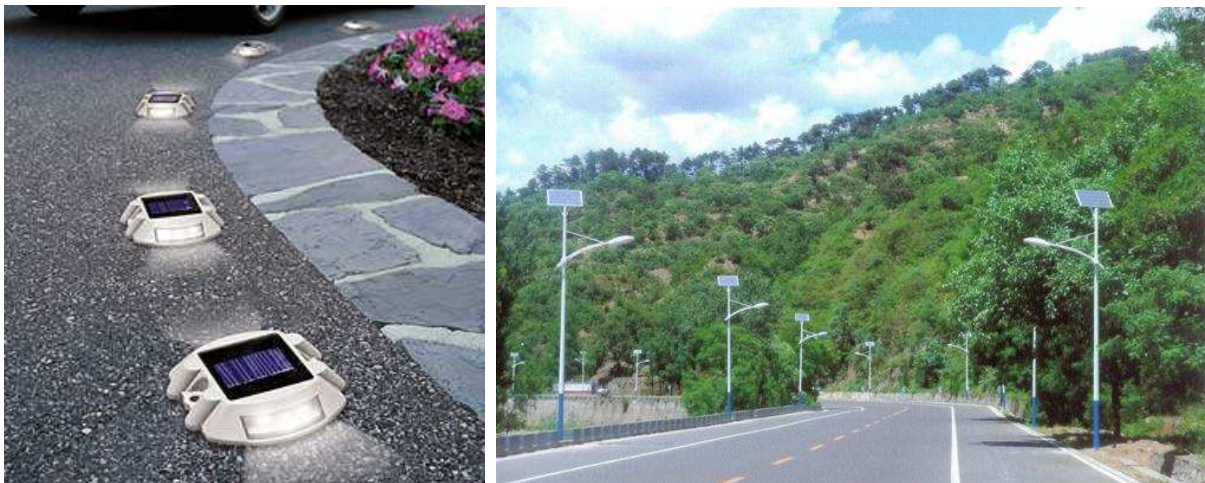
Figure 1.12: Examples of Solar Lighting: optical fibers street lights (also called "Light-Up Path" or "Spot-light") and street lamp heat lighting.
