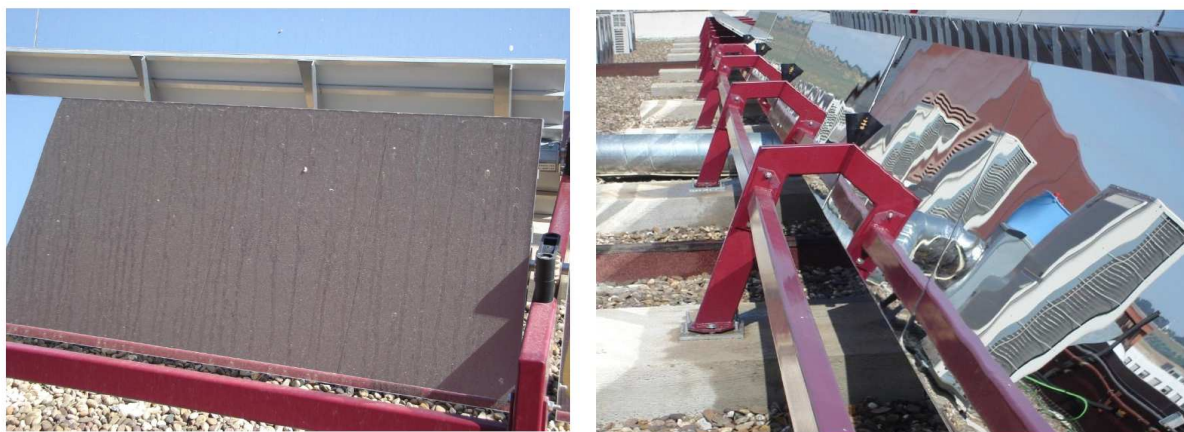
Figure 5.4: Examples of dirty mirror (on the left) and clean mirror (on the right). The parameter \alpha of the model is a cleaning index for mirrors: it is equal to 1 when mirrors are clean and its value decreases as the dirt increases.
