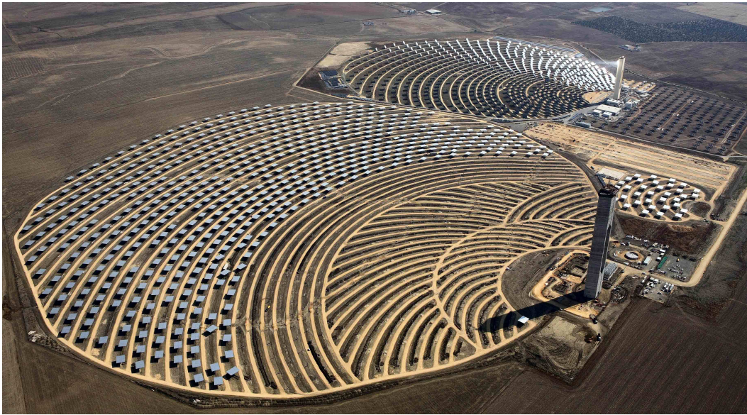
Figure 1.6: A Power Tower Plant: Stretched-membrane heliostats with silvered polymer reflectors surround the Solar Two Power Tower in Sanlúcar La Mayor, Andalusia (20km from Seville). This Plant can produce up to 23 GW per hour during all year.
