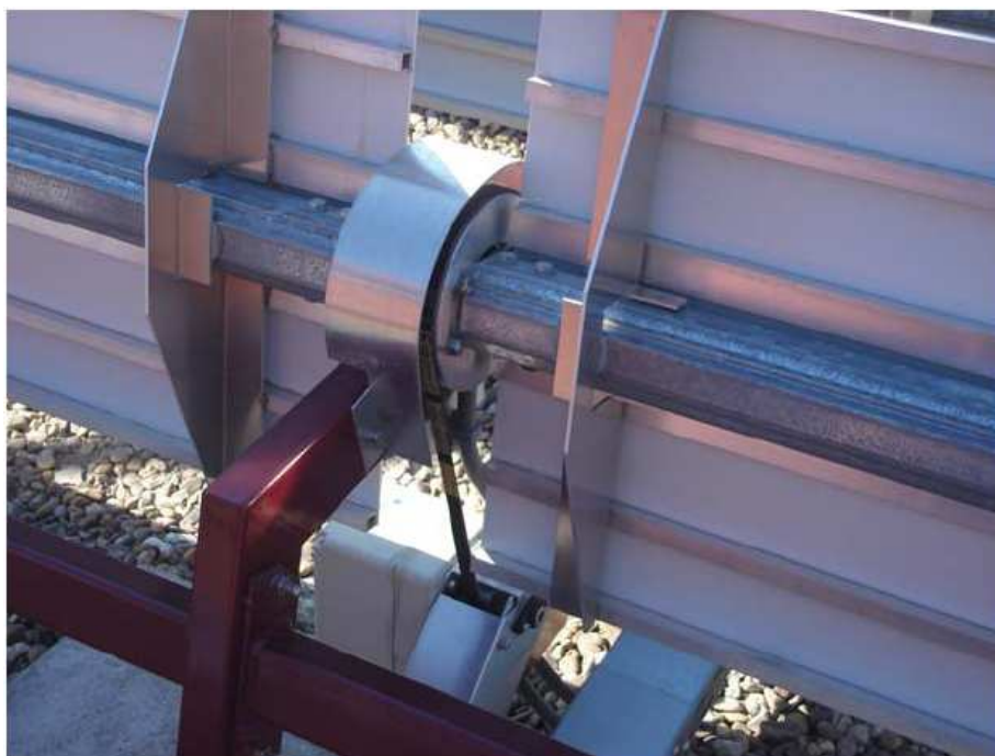
Figure 3.5: A particular of drive actuator mechanism.
