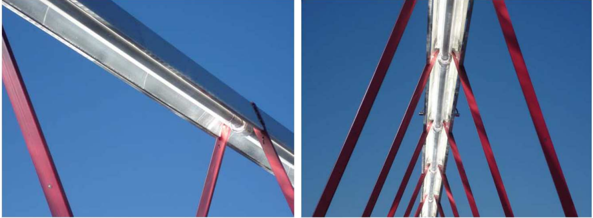
Figure 3.6: Secondary reflector (on the left) and receptor pipe (on the right).
