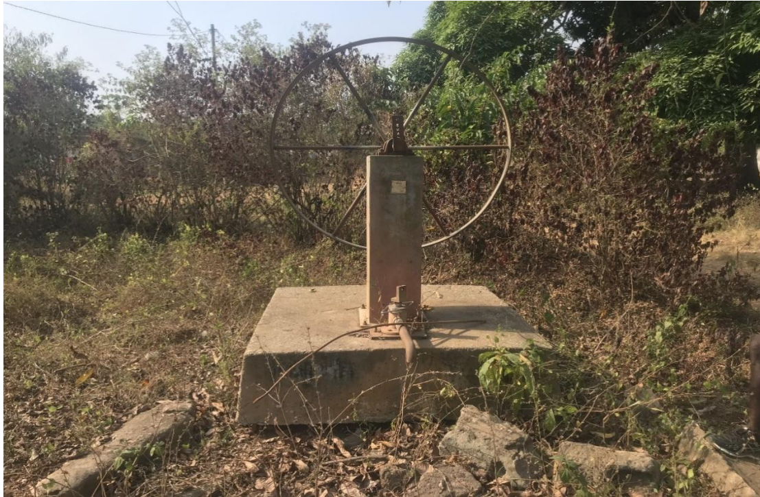
Figure 16: Abandoned VOLANTA boreholes built in the year 1990
