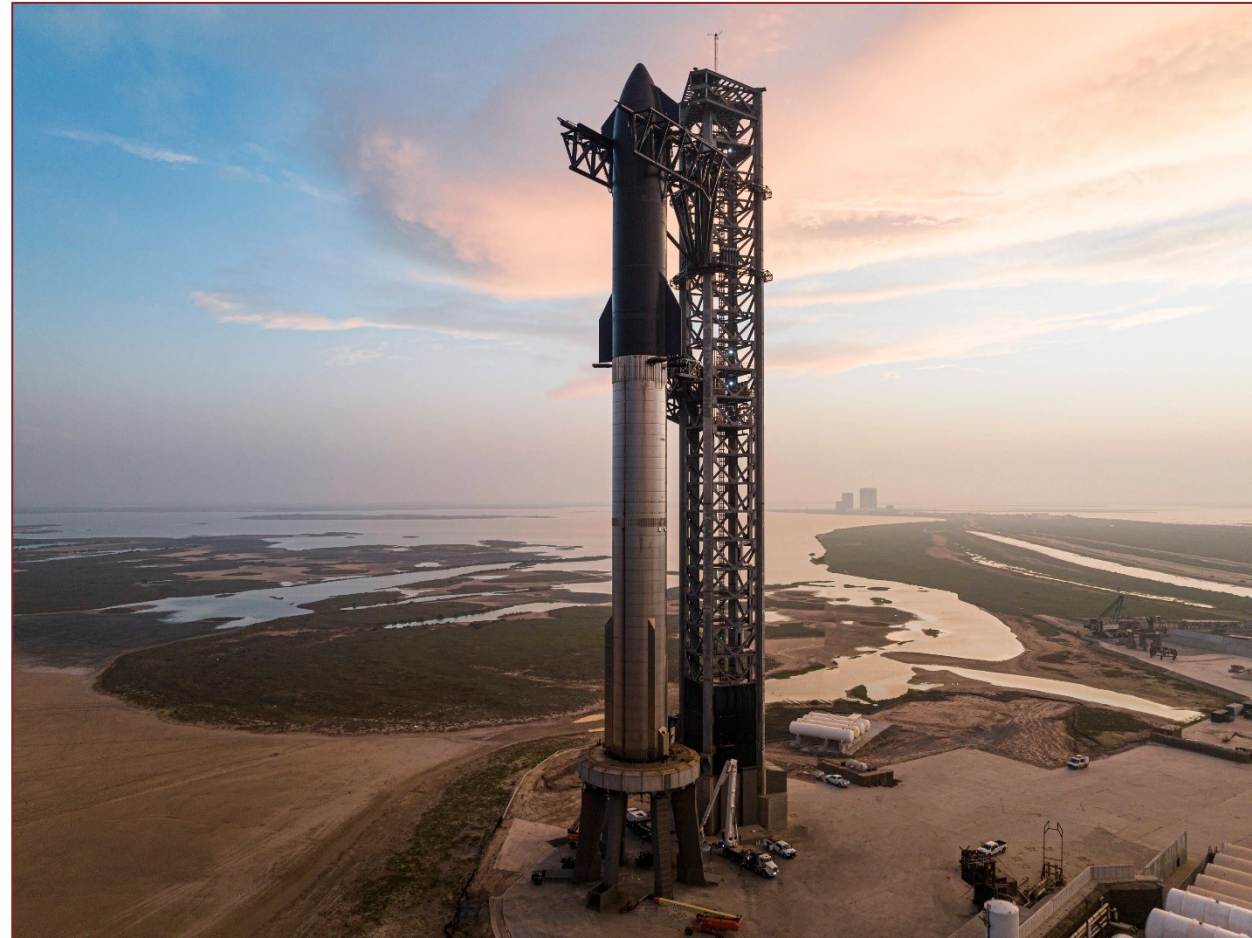
Fig.18 Starship launch facility, Texas, USA
