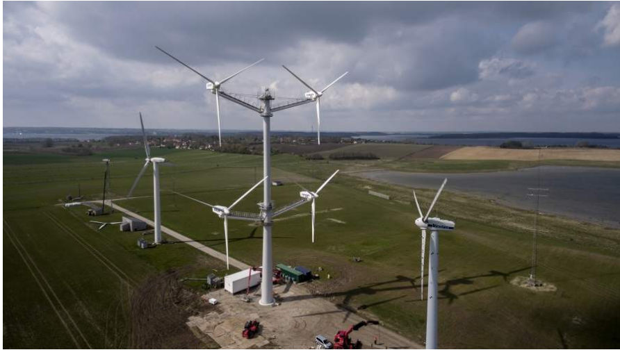
Figure 1.1: The Vestas MRT demonstrator consisting of 4 V29 225 kW nacelles and rotors. Location: DTU Risø in Roskilde Denmark. Image Courtesy Vestas Wind Systems A/S.
