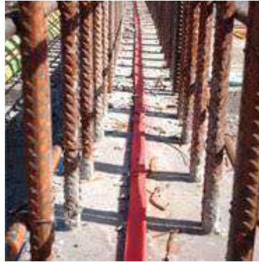
Figure 1. 29. Water stops swellable hydrophilic( www.arconsupplies.co.uk )
