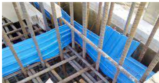
Figure 1. 28. PVC water stops seals( www.deep-jyotti.com )
