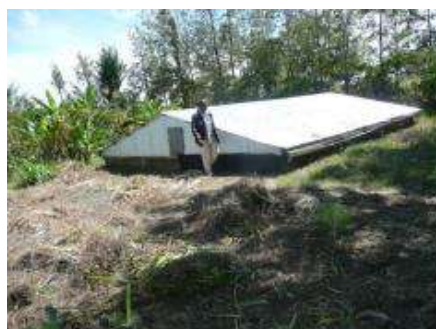
Figure 1. 15. Roofed rectangular underground tank (Bancy mati)
