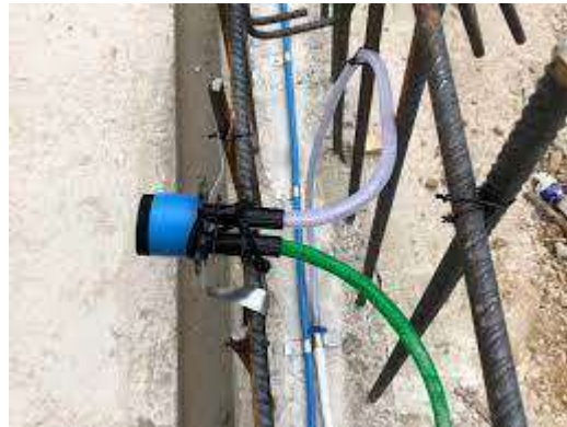
Figure 1. 31. Resin injection tube water bar( www.newtonwaterproofing.com )
