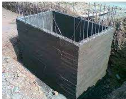
Figure 1. 4. Concrete tank( www.indiamart.com )
