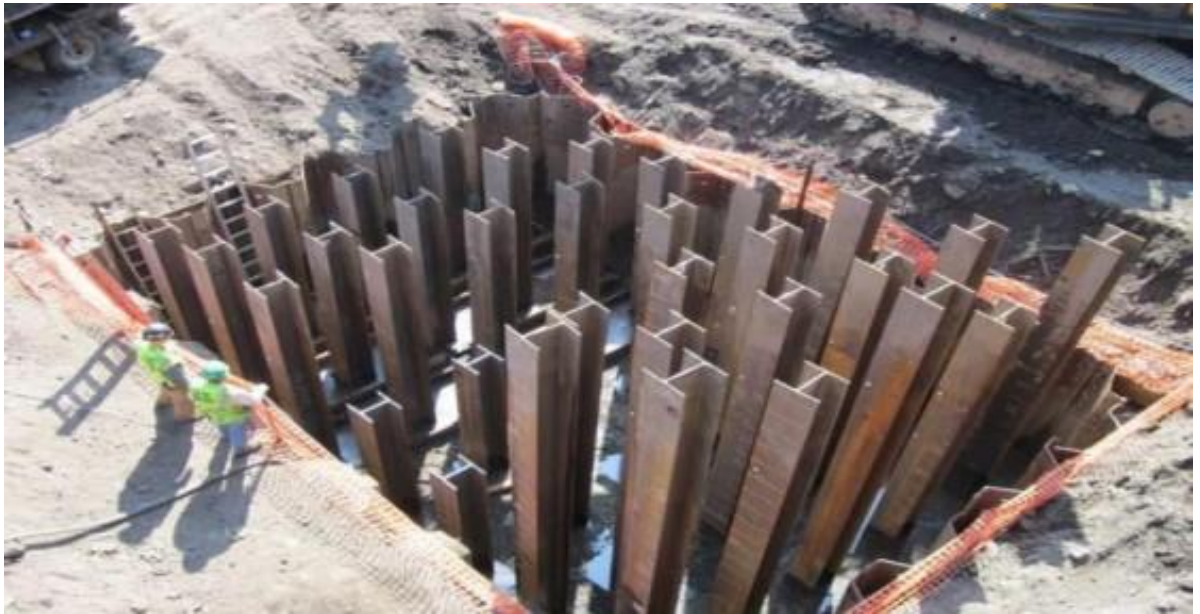
Figure 1.5. H-Steel piles (foundation blogspot.com, 24 April 2014)
