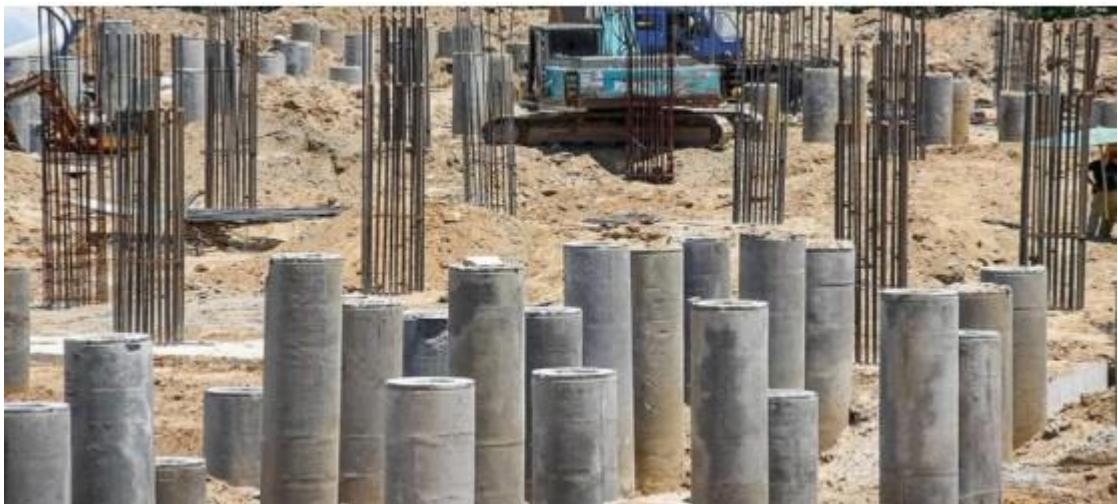
Figure 1.4. Concrete piles (www.nationalpilecroppers.com ,2021)
