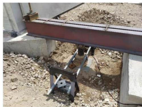
Test n.2- detail of jack and sensor positioning
