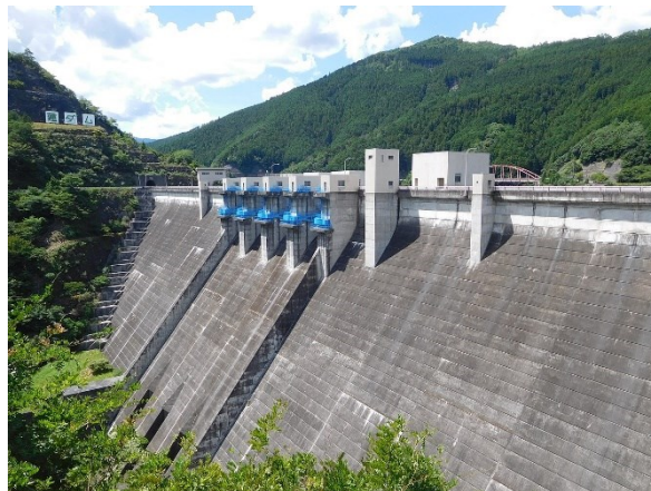
Figure 1.1: Gravity dam of Hachisu (Japan)
