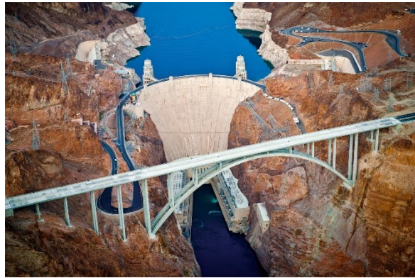
Figure 1.2: Arch dam of Hoover (USA)
