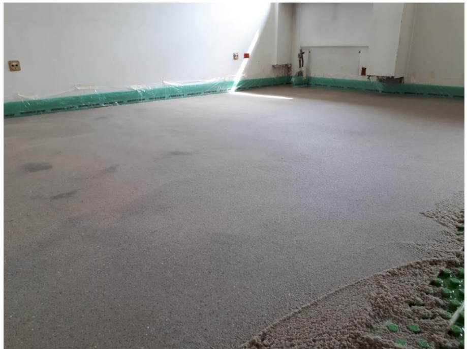
Fig. 23. Surface resin coating (screed)
