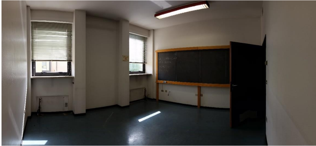
Fig. 11. Picture of the room 52 before the beginning of works
