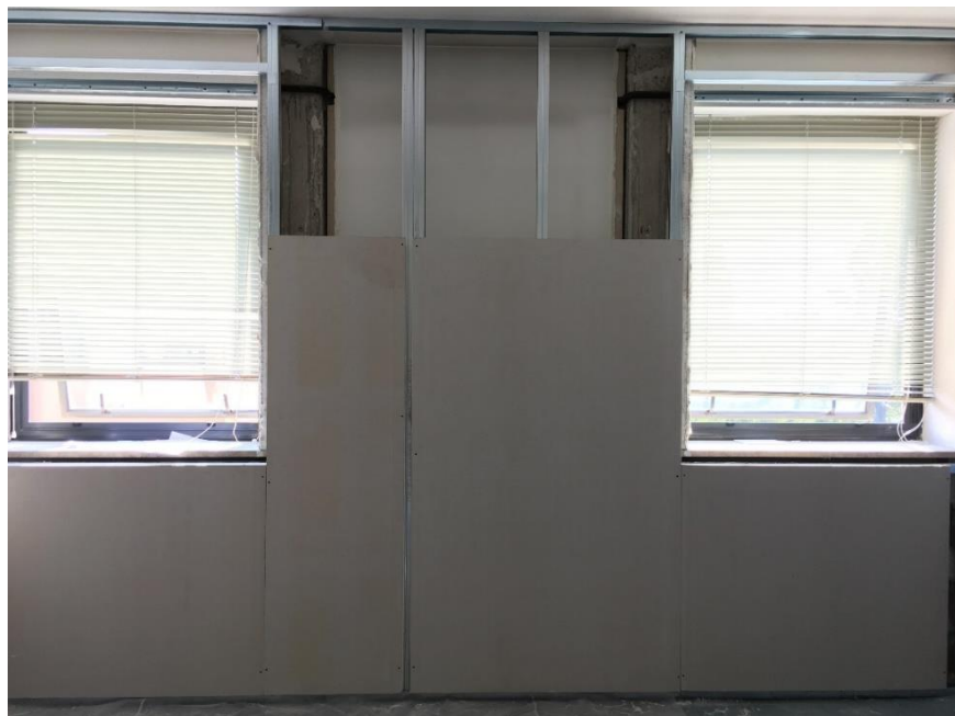
Fig. 35. East panels after the installation
