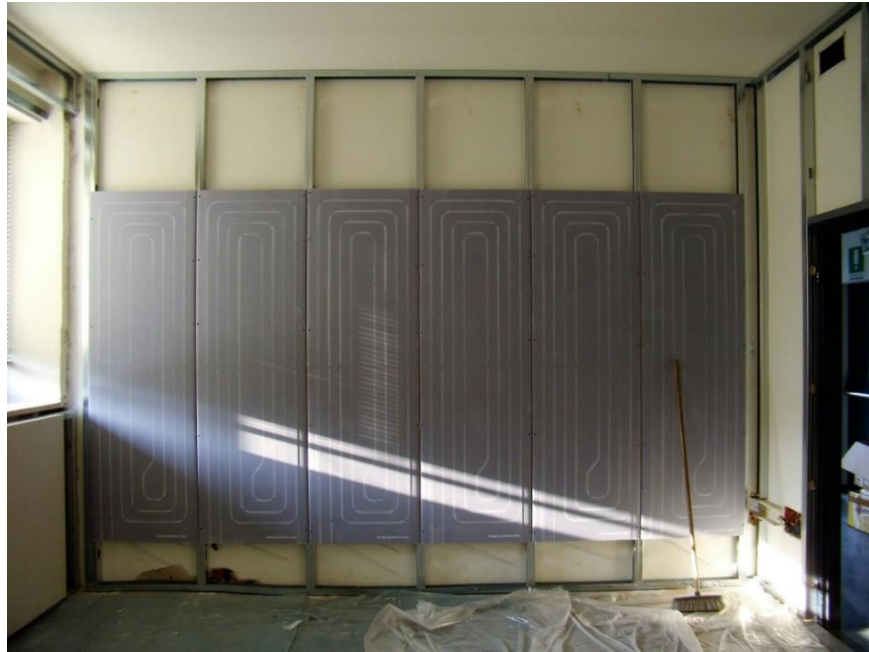
Fig. 37. South panels after the installation
