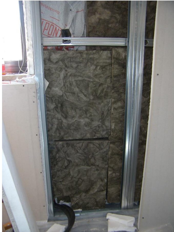
Fig. 34. Insulating material (rock wool) inside niches
