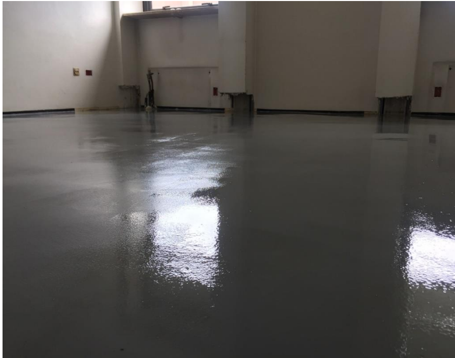
Fig. 24. Surface coating drying
