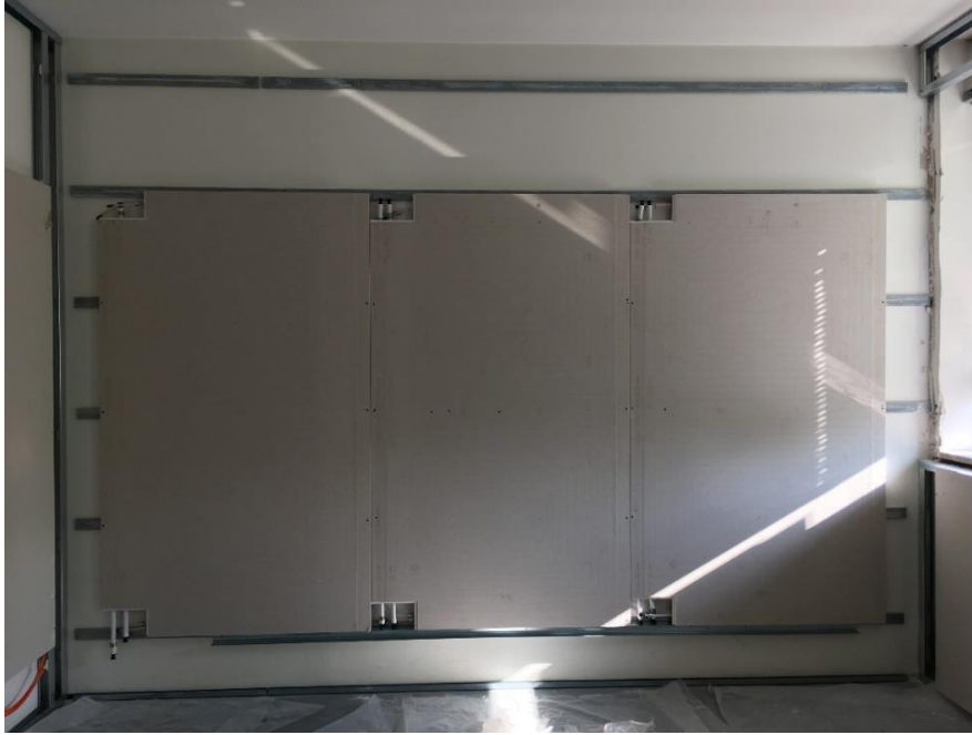
Fig. 29. North panels after the installation
