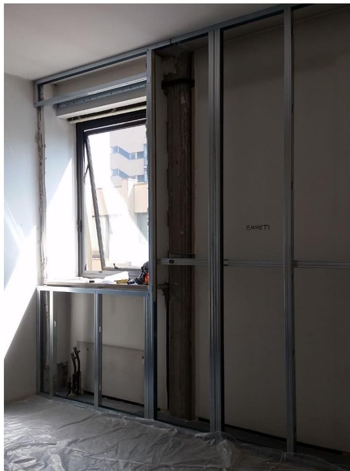
Fig. 33. Metal substructure necessary to close the existing niches
