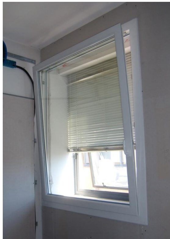
Fig. 50. One of the two windows installed in the test room
