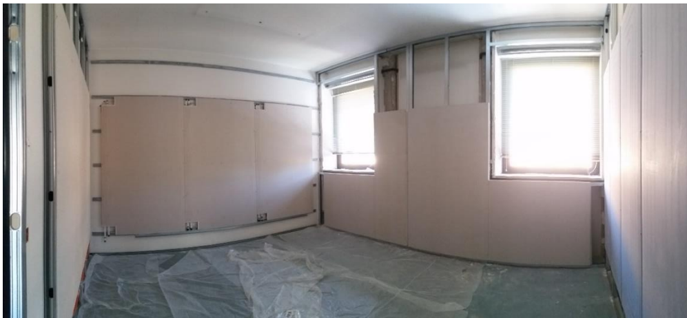
Fig. 51. North and east wall after the installation of radiant panels
