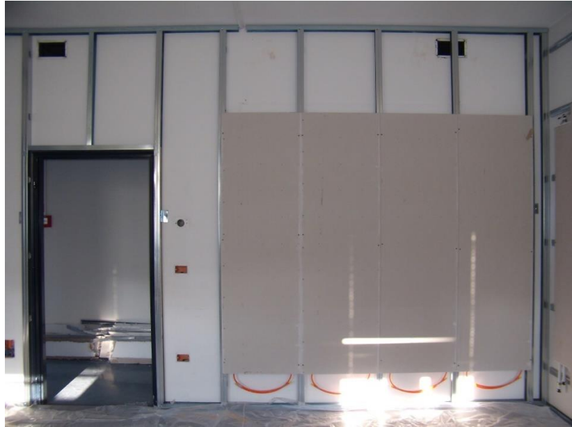
Fig. 41. West panels after the installation
