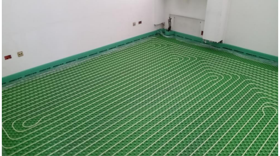
Fig. 22. Laying of panels and circuits
