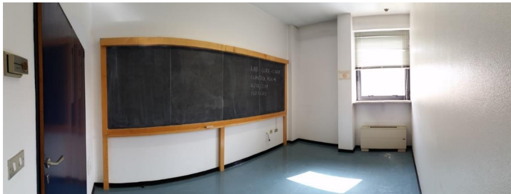
Fig. 12. Picture of the room 53 before the beginning of works
