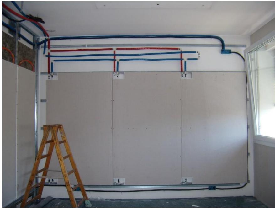
Fig. 30. North panels during the hydraulic and electrical connection
