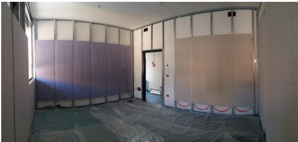
Fig. 52. South and west wall after the installation of radiant panels
