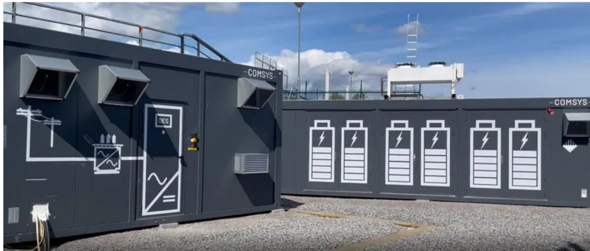
Landafors hydropower plant storage system
