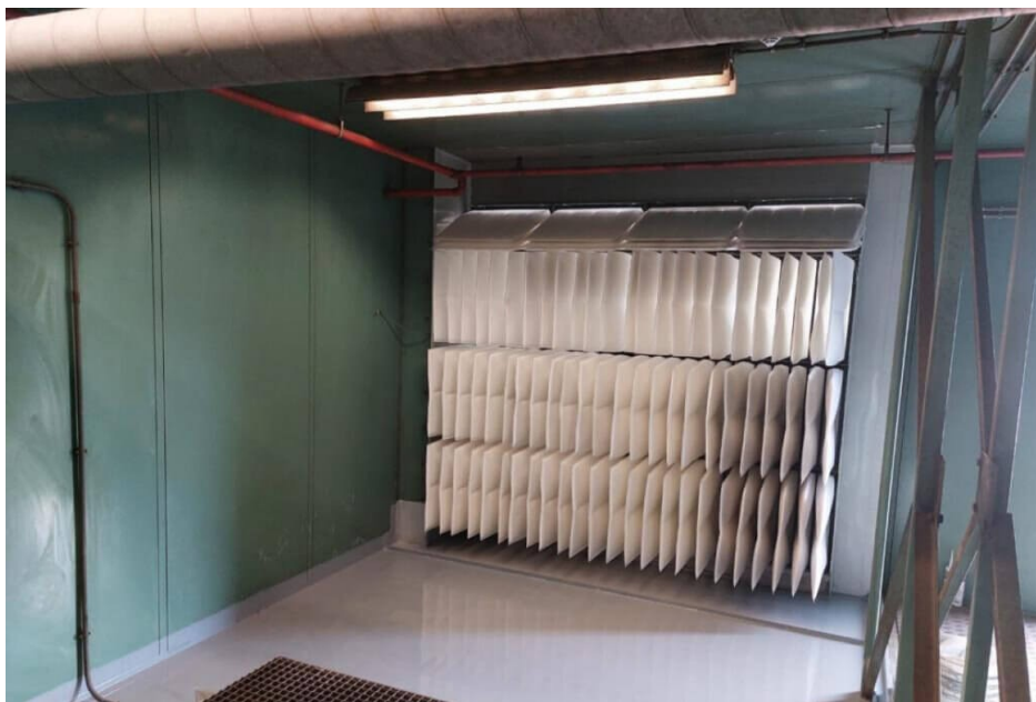
Figure 2.4: V-shape pocket filter
