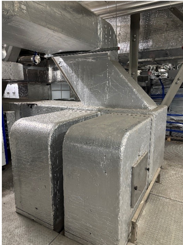
Figure 2.7: Insulated duct
