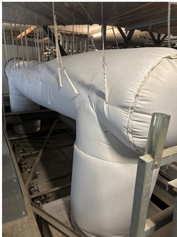
Figure 2.6: Textile duct
