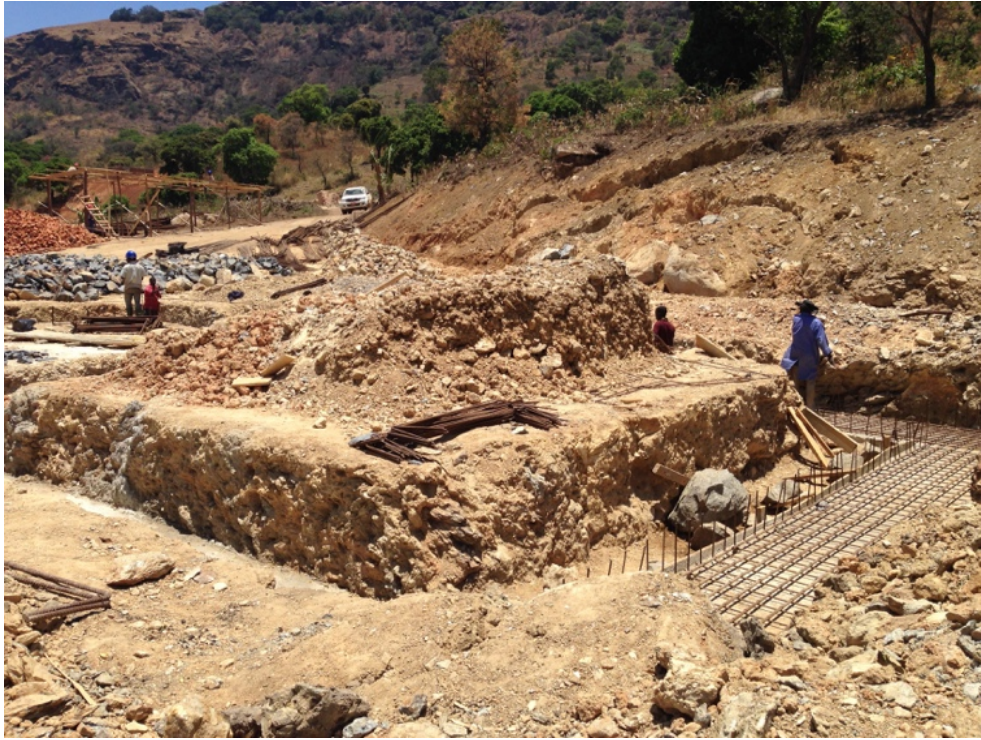
Figure 20 Powerhouse during the month of October
