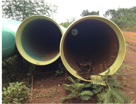
Figure 17 Pipes of the penstock
