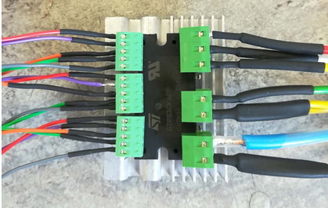
Figure 10.1: Inverter pins popped into the connectors
