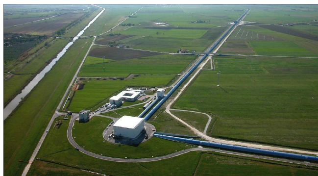
Figure 1.4: Aerial view of the Virgo detector (image credit: The Virgo Collaboration).
