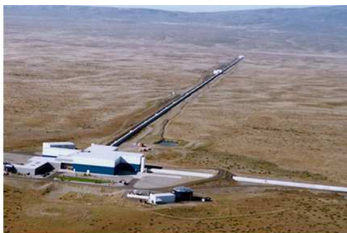
Figure 1.3: Aerial photograph of the LIGO observatory at Hanford, Washington. The laser and optic is contained in the large corner buildings, where beam tubes extend for 4 km in each direction. The tubes are covered by the arched, concrete enclosures. Image from [9]
