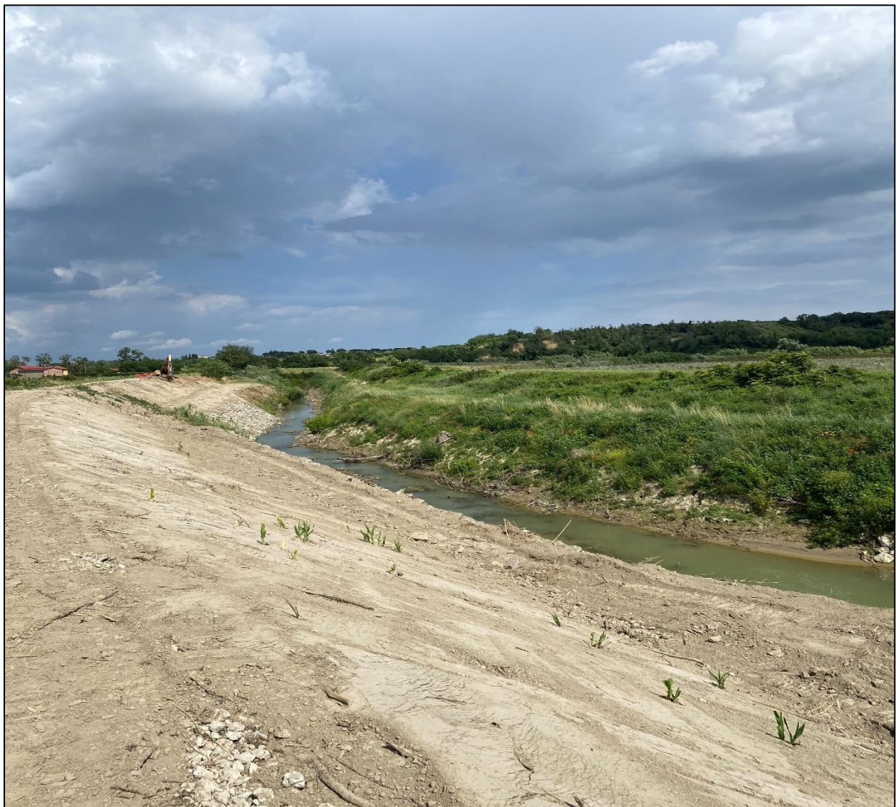
Figure 4.10: Intervention works at Via Canale breach, June 03, 2024 site inspection
