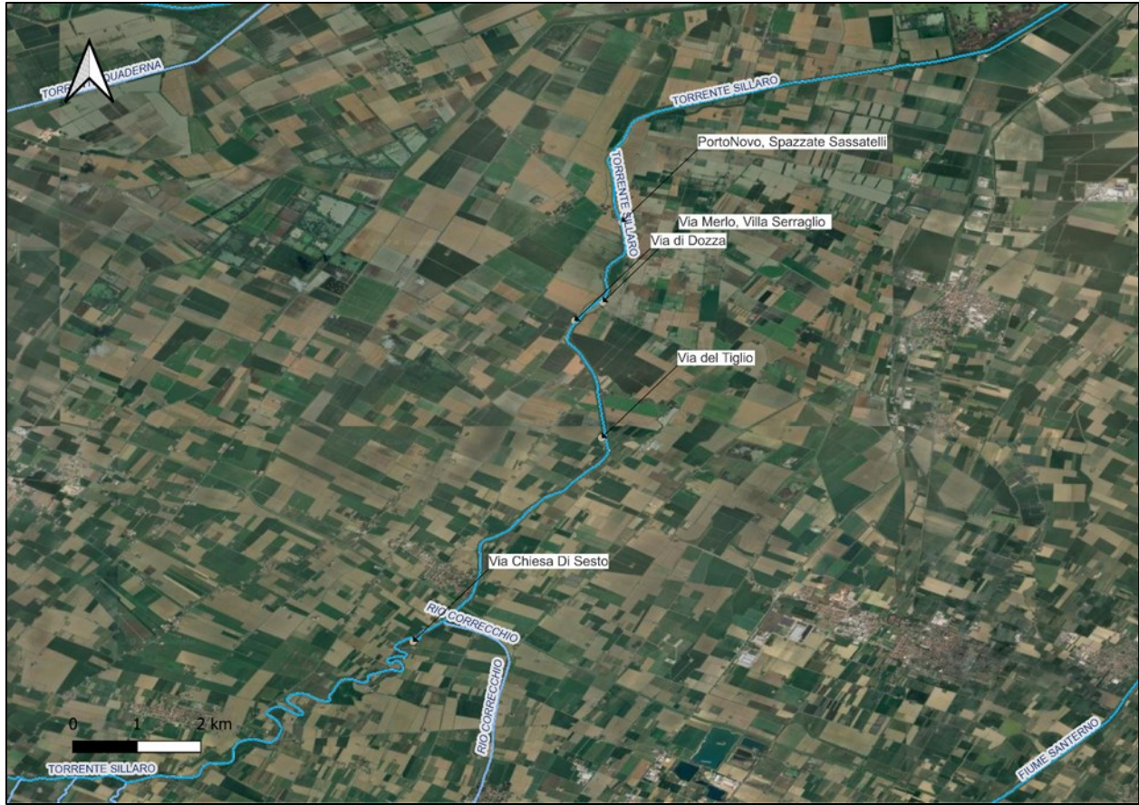
Figure 4.6: Breaches along the Sillaro watercourse
