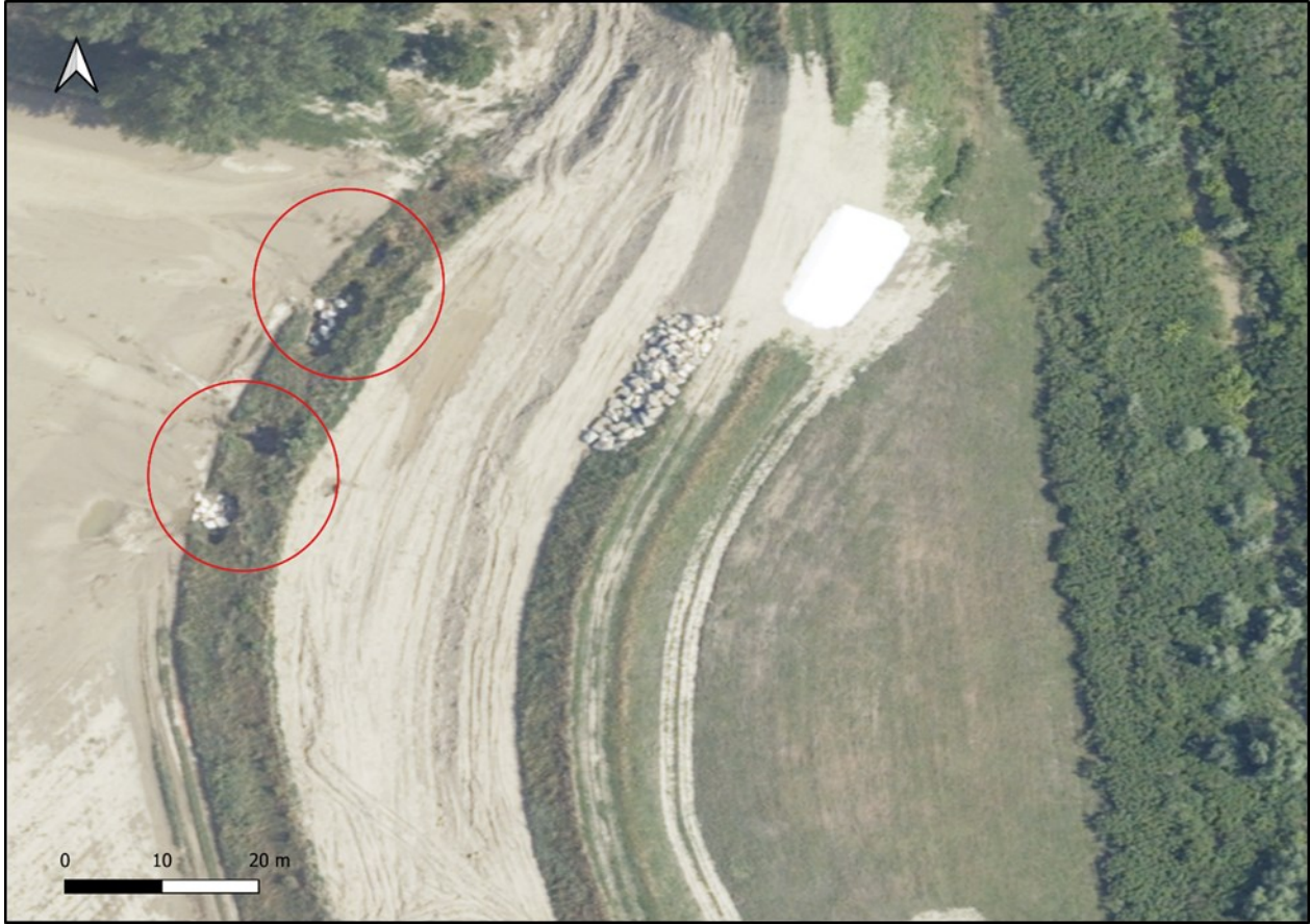
Figure 6.2: Observed possible piping sign at Sillaro River
