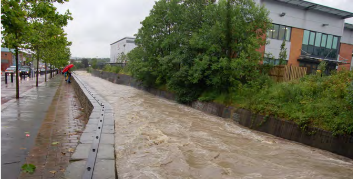
Figure 2.10: River Sheaf during 2007 flooding, Sheffield, U.K.
