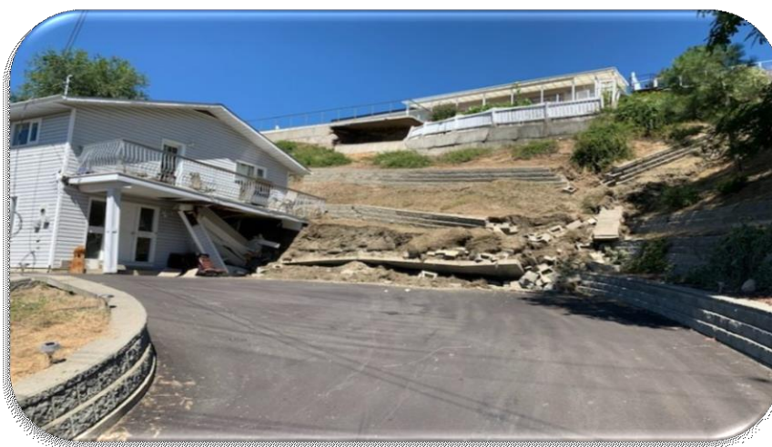
Figure 1.17. Slope stability failure (Source: civilblog.org)
