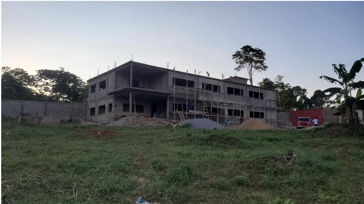
Figure 3.2. Nsimalen industrial building
