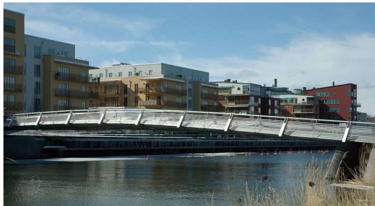
Fig. 9 Apatè bridge in Stockholm made of duplex 2205 [4]
