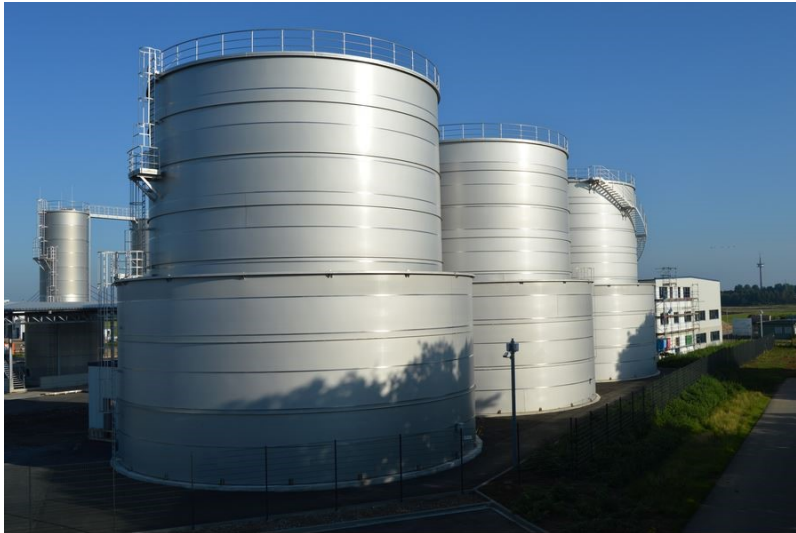
Fig. 8 Duplex storage tanks in LDX 2101 for liquids hazardous to water [18]
