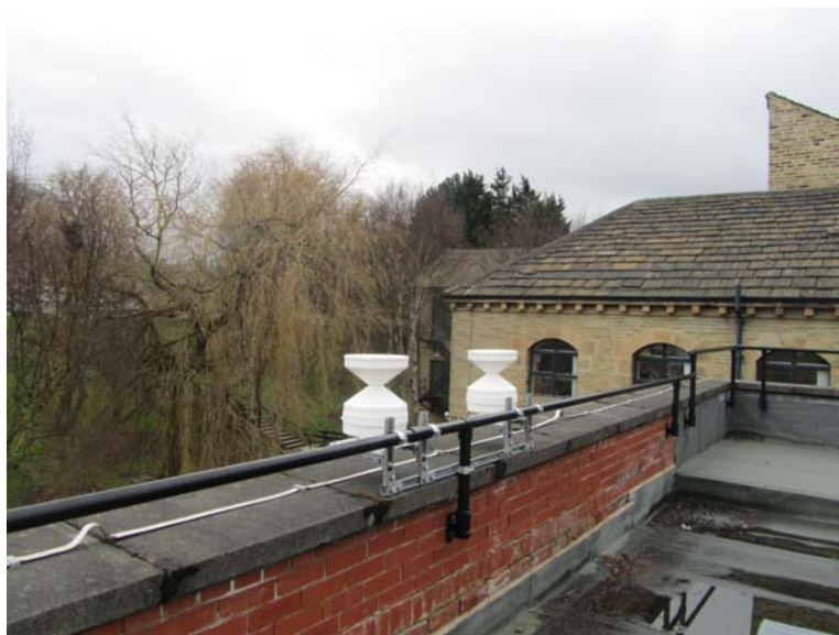
Figure 13: Rain gauges of point A, in Phoenix building.
