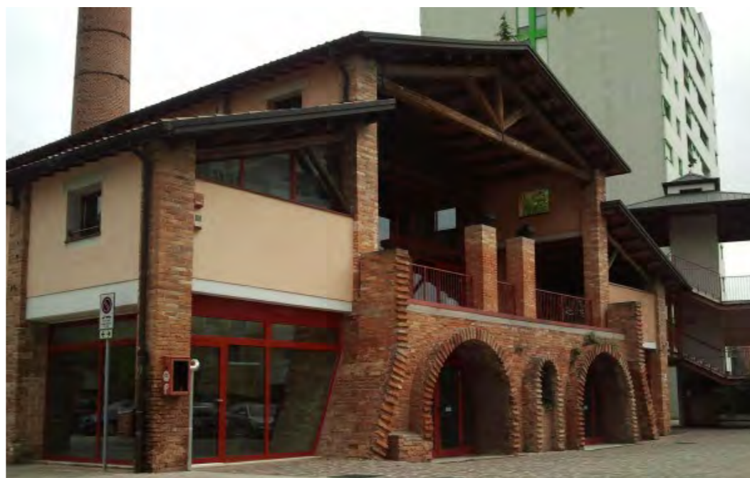
Fornace Carotta a Padova
