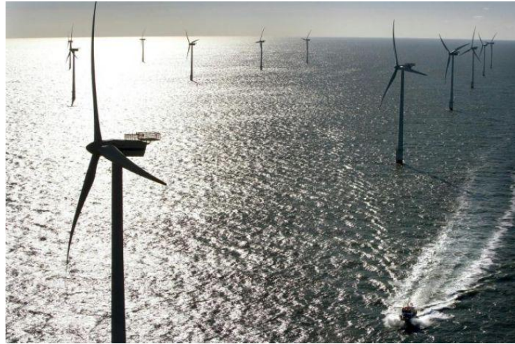
Figura 1.3 – Wind farm off-shore
