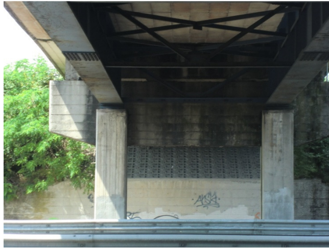
Figura 118: Pile e pulvino in c.a.
