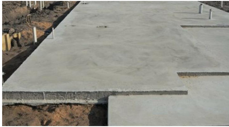
Figure 1.9. Slab on grade ( www.civilsapshot.com )
