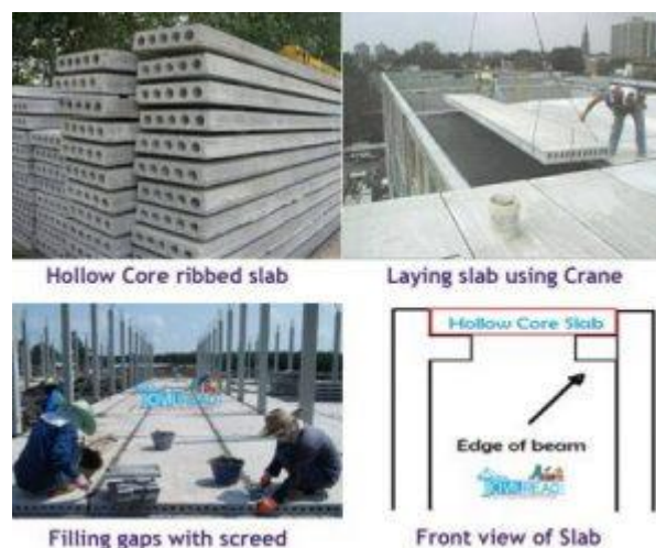
Figure 1.5. Hollow core ribbed slab (civilread.com)
