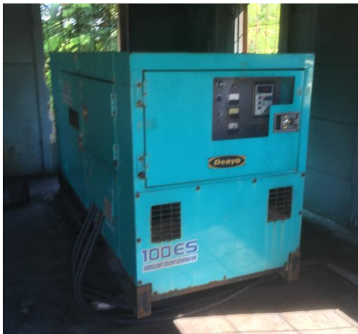
Figure 4.1 (left): The Engine-drive AC generator operating in Guasasa; Figure 4.2 (right): Diesel tank of the generator set in Guasasa (Ciemat, 2020).
