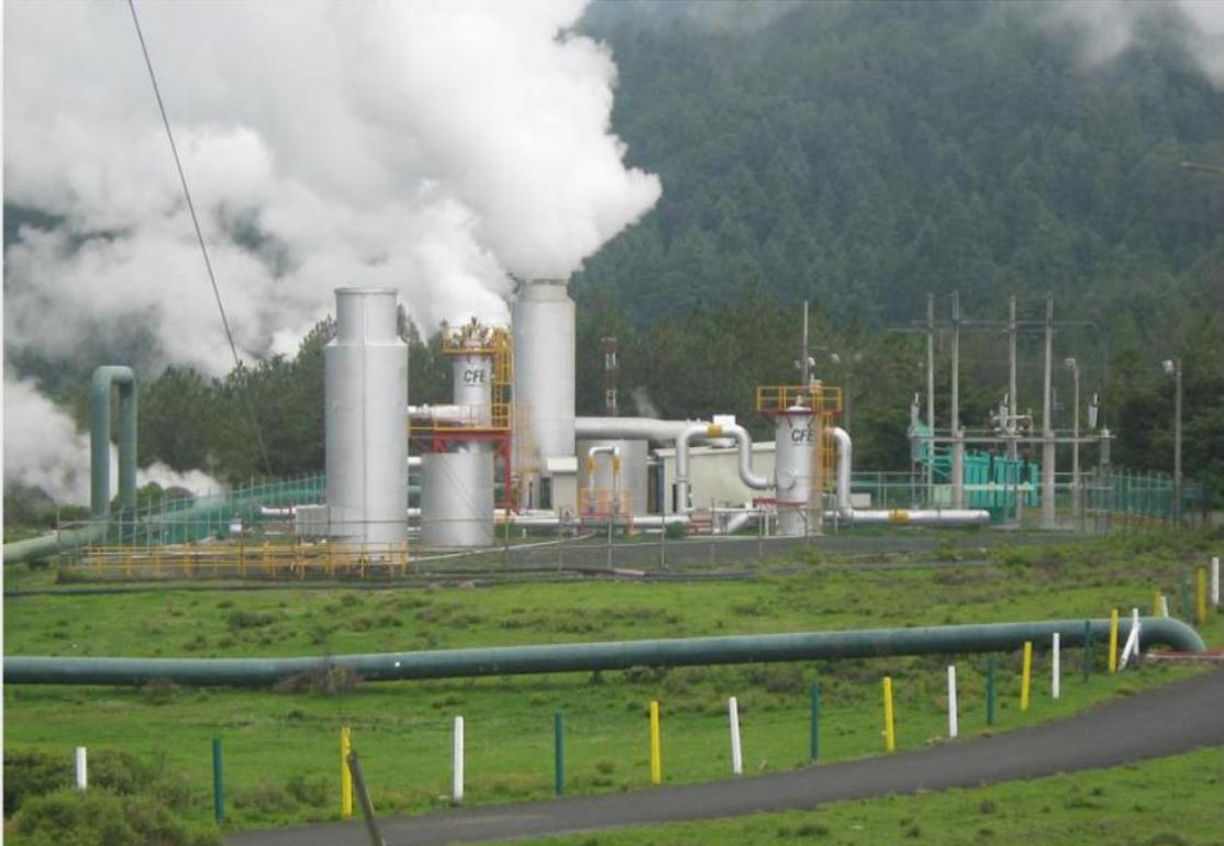
*Figure 17: Unit 3, located in the north zone of LAGF, producing 5 MW of electrical energy, to be dismantled in 2015.*
