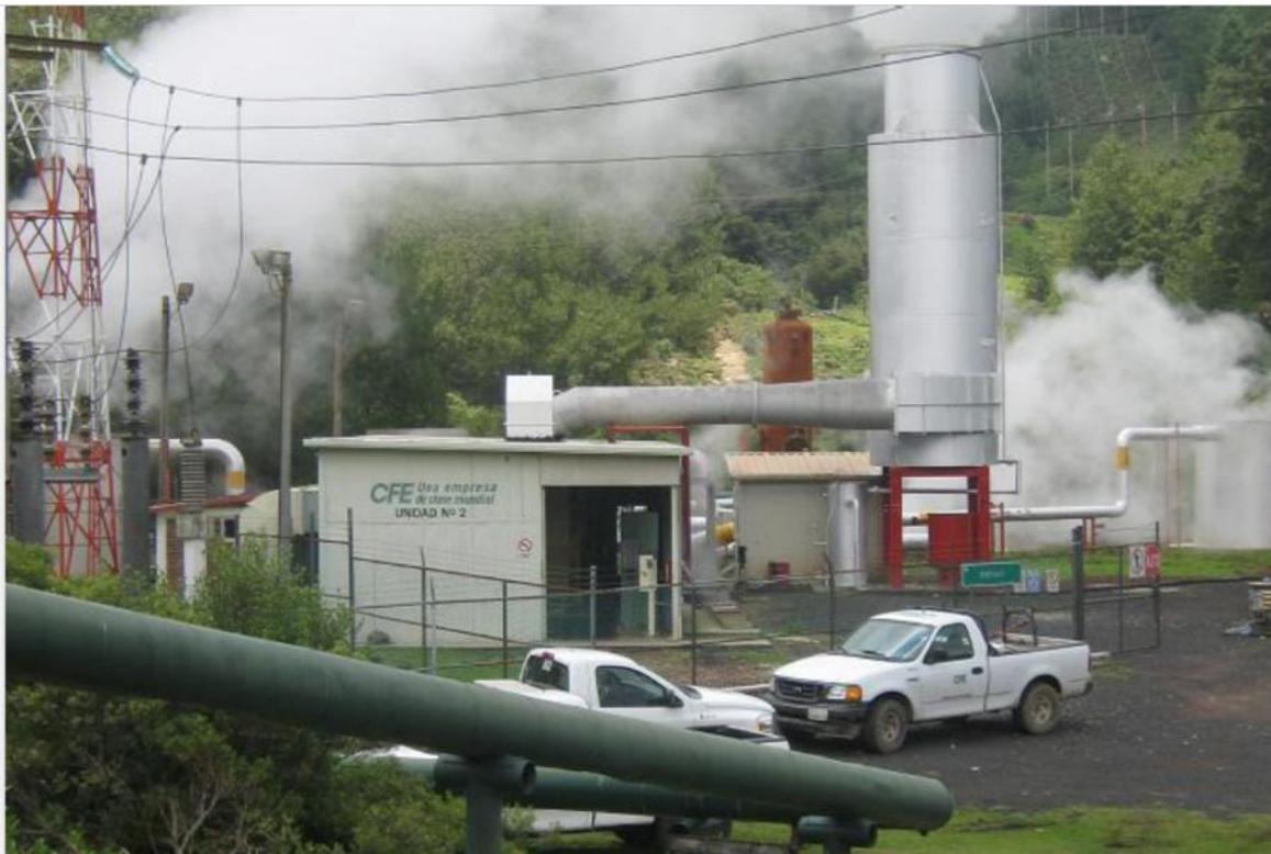
*Figure 16: Unit 2, located in the south zone of LAGF, producing 5 MW of electrical energy, to be dismantled in 2015.*
