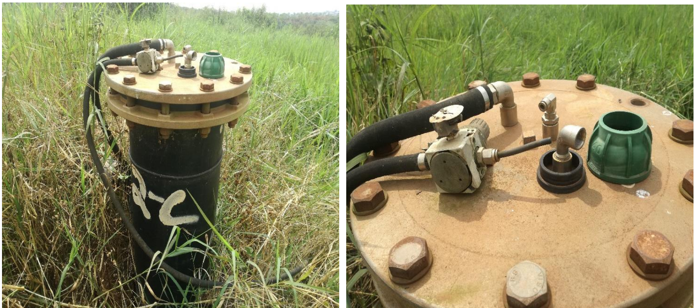
Fig 11: An example of a mixed well with manometer and pneumatic pump
