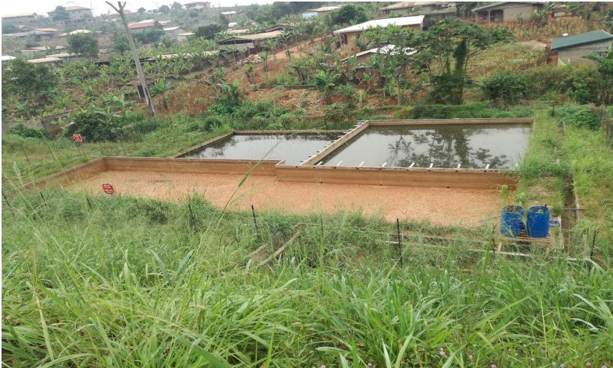
Fig 11: Leachate flow in landfill: a) leachate flow by gravity; b) lagoon (3,5 m deep) c) Leachate treatment basins (Three compartments with volumes of 180 m 3 capacity)
