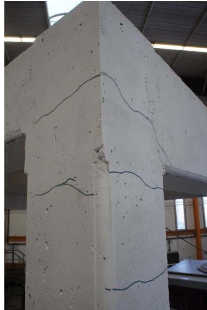
Figure 6.29: 2 nd floor beam-column joint before test sequence 1 (Garcia et al. 2012)
