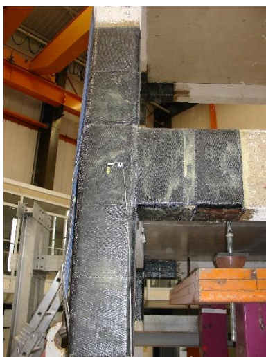
Figure 4.5: CFRP strengthening in 1 st floor (Garcia et al. 2012)
