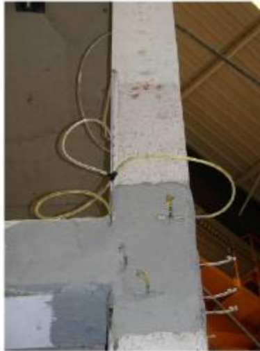
Figure 2.16: Epoxy resin injection in a damaged joint (Bandit Project 2012)
