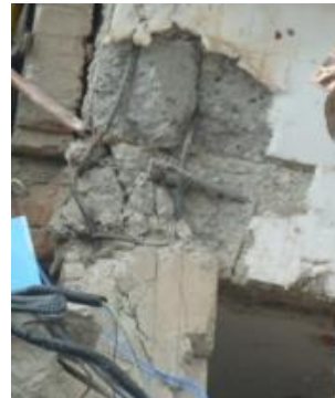
Figure 2.3: RC building in Cavezzo (MO) Emilia Romagna, 2012
