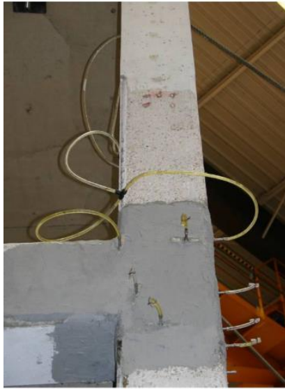
Figure 4.3: Epoxy resin injection in a damaged joint (Garcia et al. 2012)
