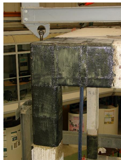
Figure 4.6: CFRP strengthening in 2 nd floor (Garcia et al. 2012)
