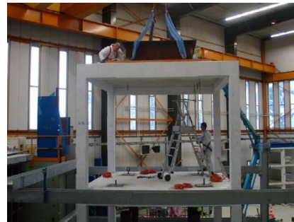
Figure 3.3: Clamping of the masses on the second slab (Garcia et al. 2012)
