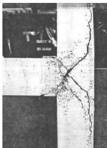
Figure 2.12: Exterior joint specimen exhibits Damage State 9
