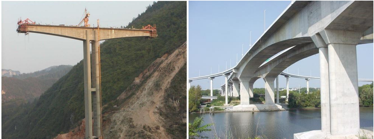
Figure 6.27: Two examples of balanced cantilever method.
