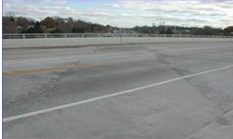
Figure 3.25: ECC link slab in a bridge in Michigan [6].
