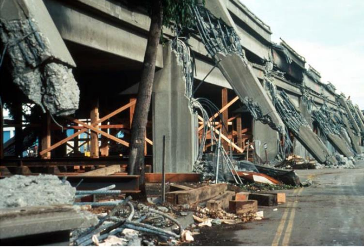
Figure 2.2: Cypress Street Viaduct of Interstate 880 [2].
