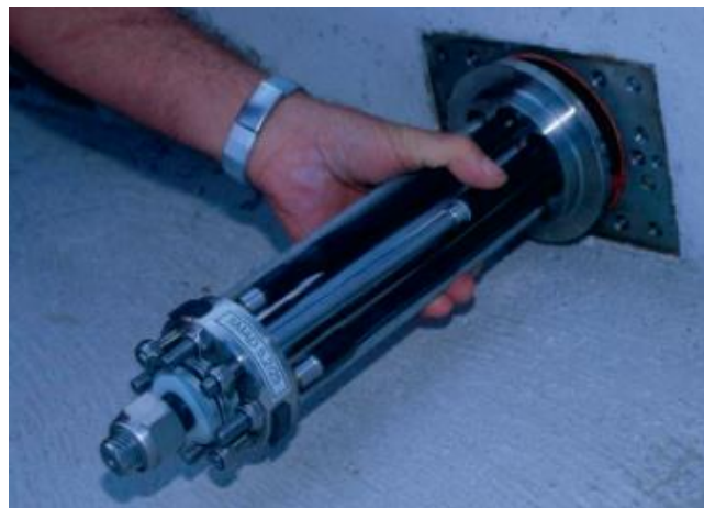
Figure 4.17: Basilica of San Francesco in Assisi's SMA device [7].
