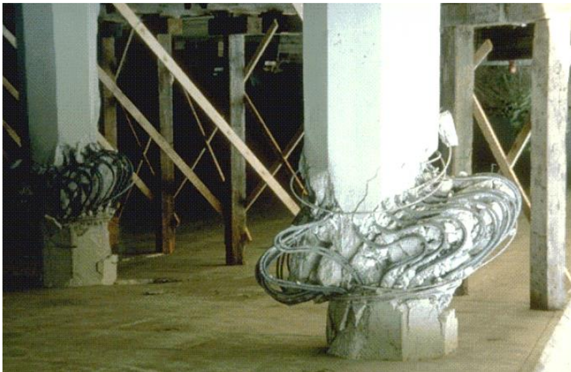
Figure 2.5: RC columns under the Valley Freeway in 1994 [2].
