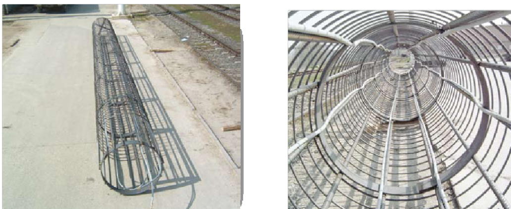
Figura 11: pilastrini energetici (Rehau S.p.a., 2007)
