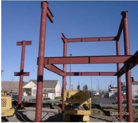
Figure 3.15: Shop-Fabricated CFT Joint
