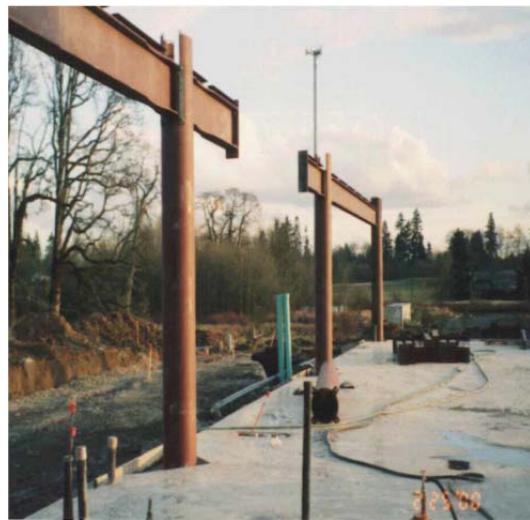
Figure 3.13: Field-Fabricated CFT Joint
