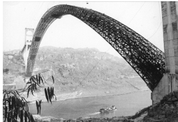
Figure 3.10: Arch Rib Being Erected
