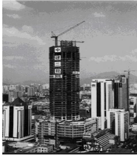
Figure 3.11: SEG Plaza under Construction in Shenzhen, (China)
