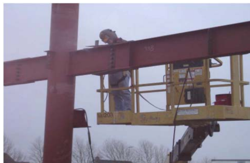
Figure 3.16: Girder Connection for Shop Joint
