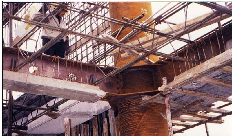
Figure 3.9: Two Direction Dense Ribs Story System
