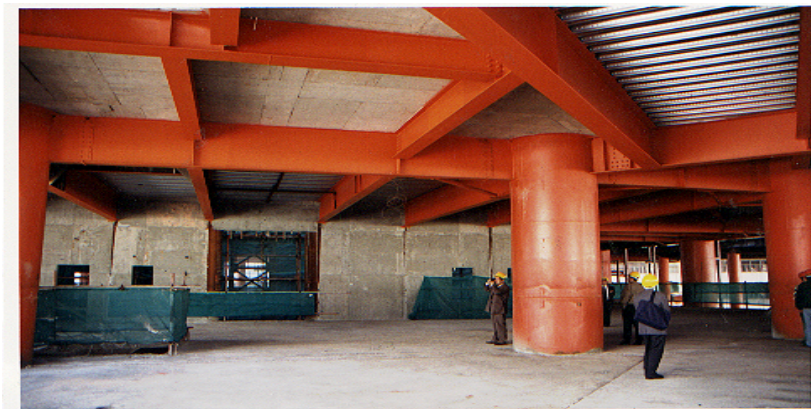
Figure 3.8: Composite Steel Story System
