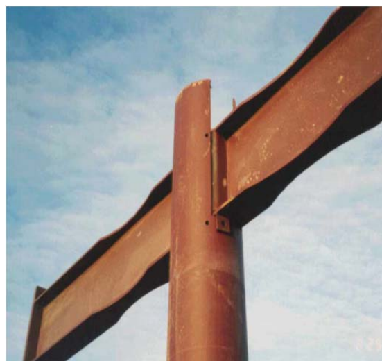
Figure 3.14: Bent Plate Closure on Girder Web
