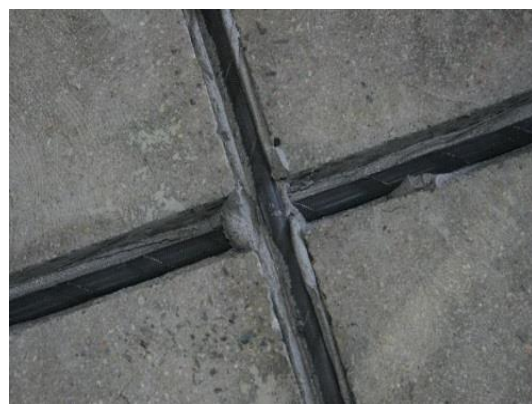
Figure 1.2. Bonding external carbon fibers bars.
