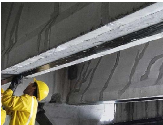
Figure 1.1 Externally-bonded laminates.
