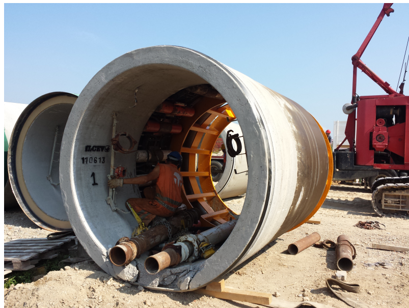
Figura 23 Intermediate Jacking Station .
