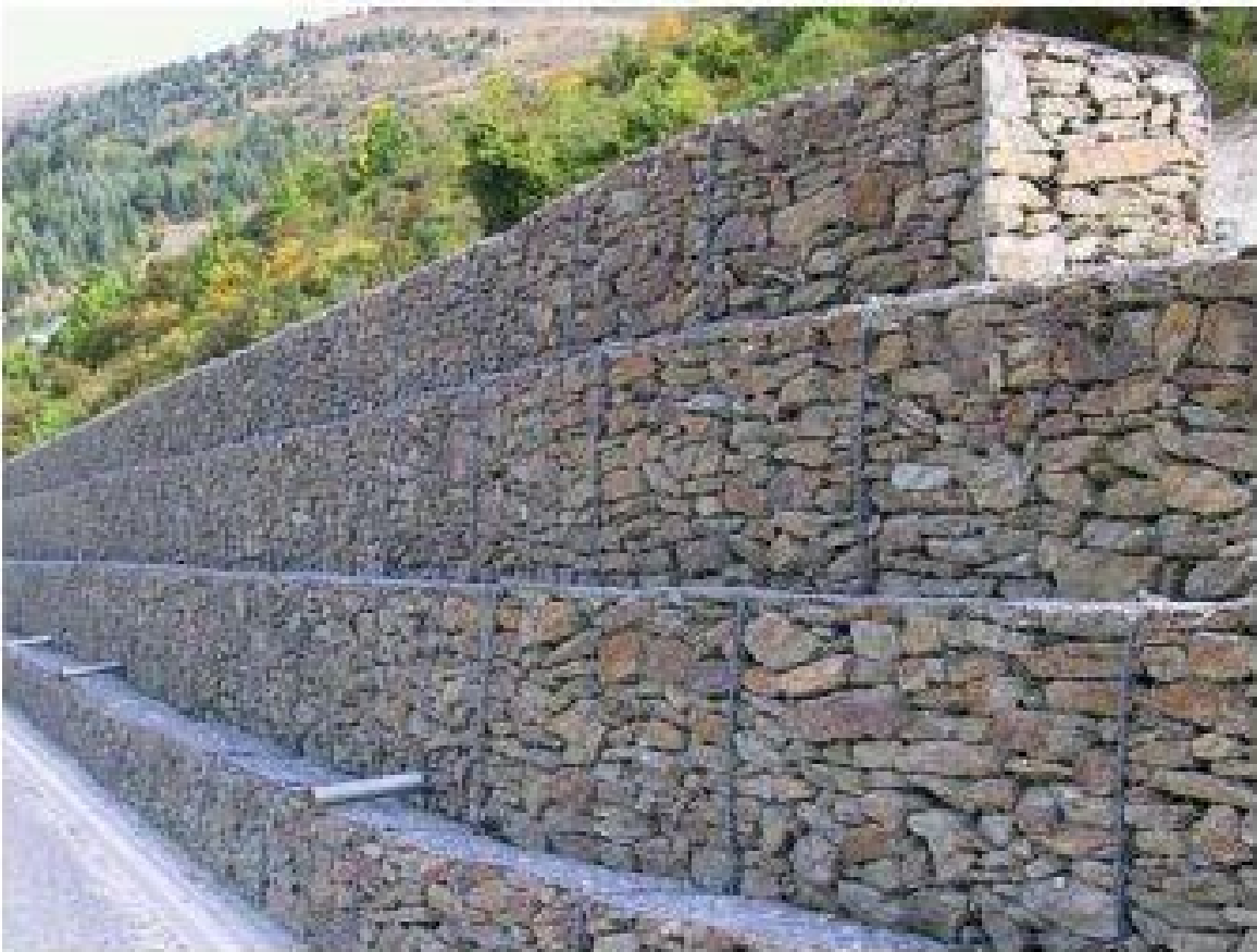
Figure 1.20. Example of a Gabion wall (Bizimana & Sönmez, 2015)
