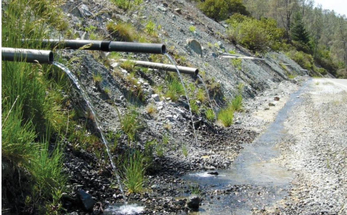
Figure 1.19. Schematic of drainpipes(Highland & Bobrowsky, 2008)
