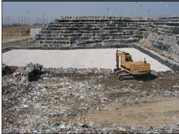
Fig. 2.5 – Daily coverage on the active edge
