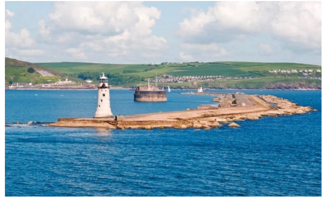
Figure 1.2. Plymouth breakwater, England. (cryllacottages.co.uk)
