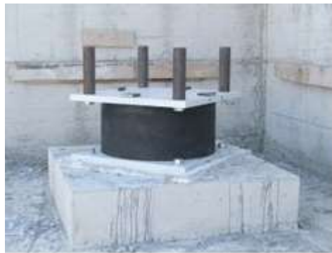
Figure. Example of seismic insulation system.
