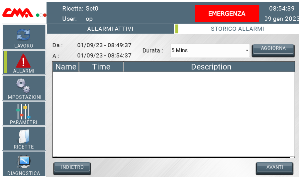
Figure 3.14: Alarms history page of the operator panel
