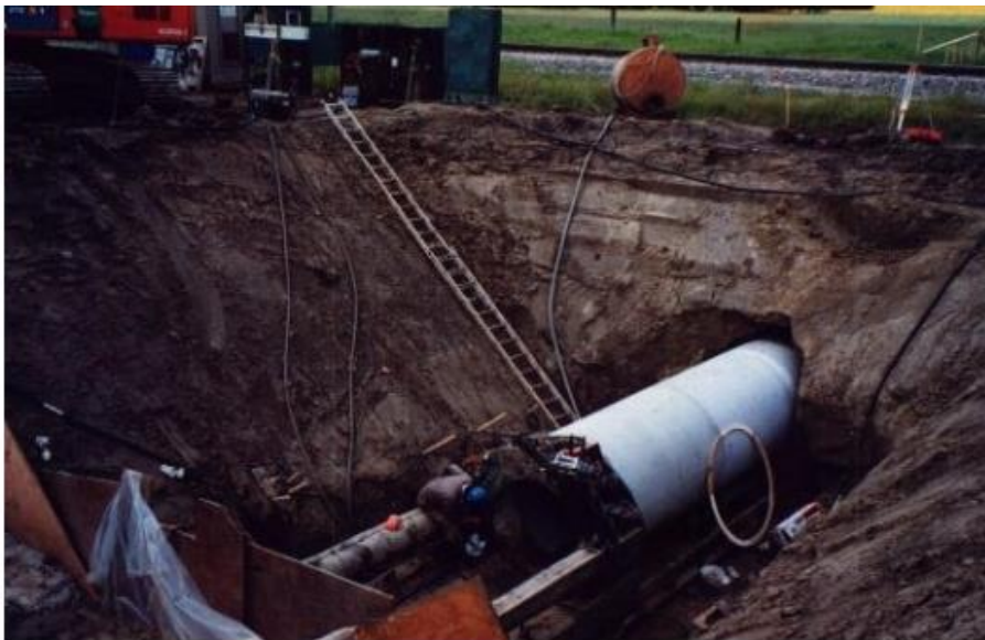
Figure 1.12. pipe jacking (Tunnel construction techniques and their details Article ,2020)
