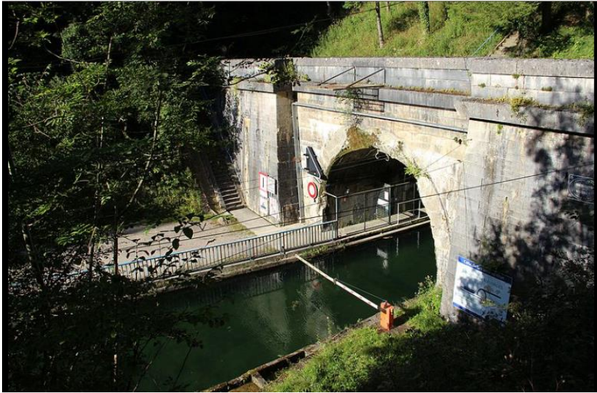
Figure 1.3 . Entrance to the Mauvages tunnel
