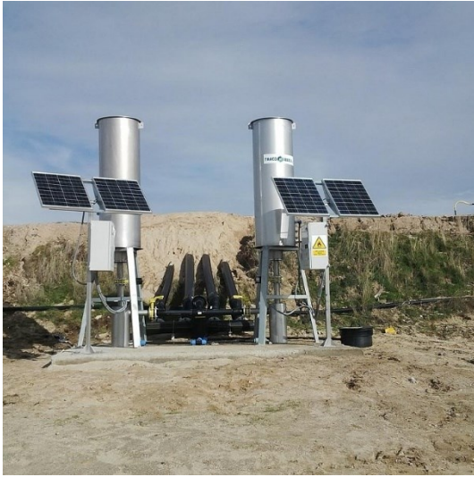
Figure 3.7 Static flares (left) and high-temperature flare (CONVECO SRL, 2022)
