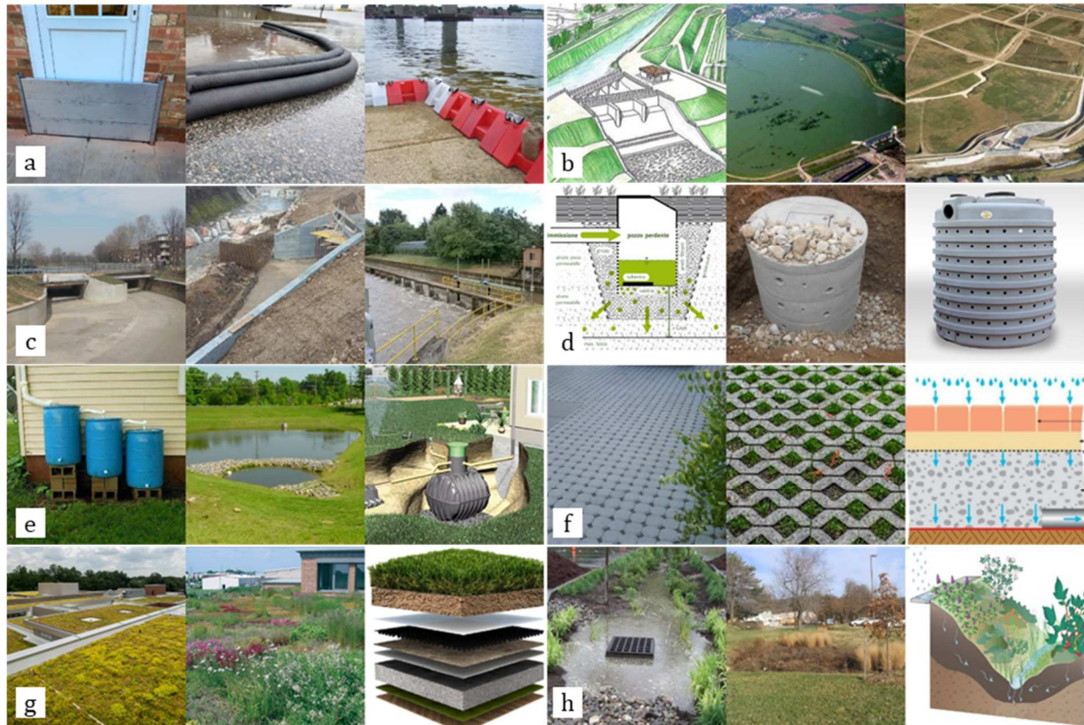
Figure 3 Examples of the water management systems presented in the survey: a) temporary flood barriers; b) expansion basins; c) diversion channels; d) soakaways; e) rain harvesting systems; f) pervious pavements; g) green roofs; h) bioretention systems.
