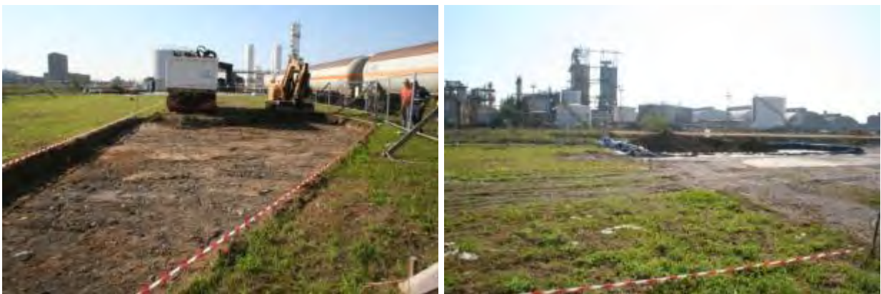
Fig. 7.1.2 Excavation and temporary disposal operations on VP_38 site.
