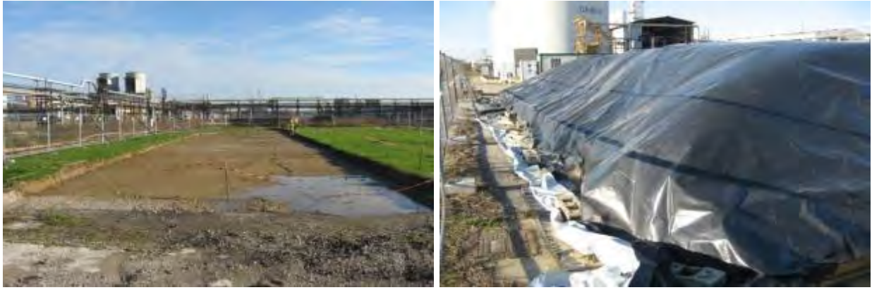
Fig. 7.1.3 Excavation and temporary disposal conclusion on VP_38 site
