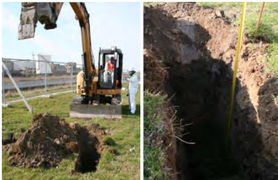
Fig. 7.7.2.3 Trench digging and depth measuring procedure.
