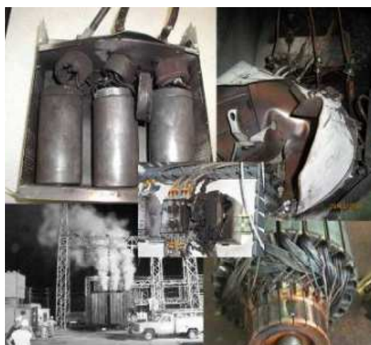
Figure 1.6. Common damages on transformers and motors
