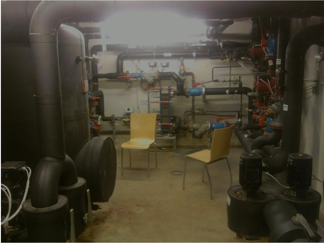
In the image above it can be seen the mechanical room, with all pipes, pumps and valves that are insulated to minimize circulation heat losses. The expansion vessel in the image down here.
