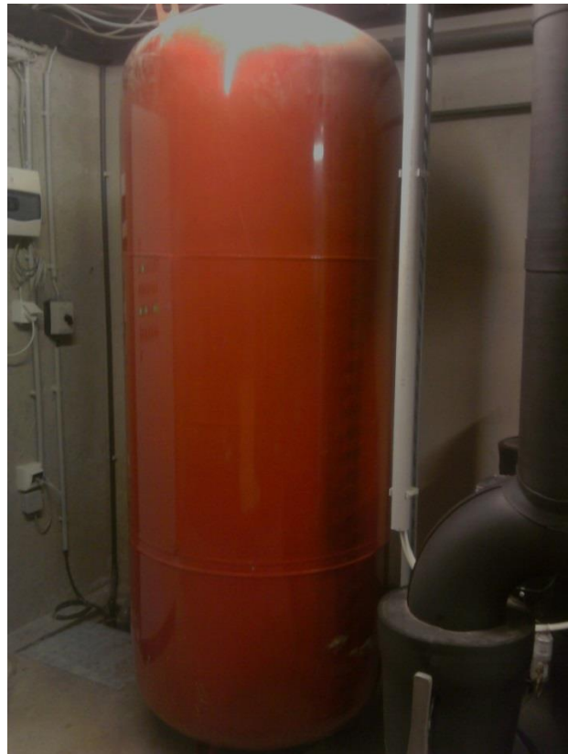
In the image above it can be seen the mechanical room, with all pipes, pumps and valves that are insulated to minimize circulation heat losses. The expansion vessel in the image down here.
