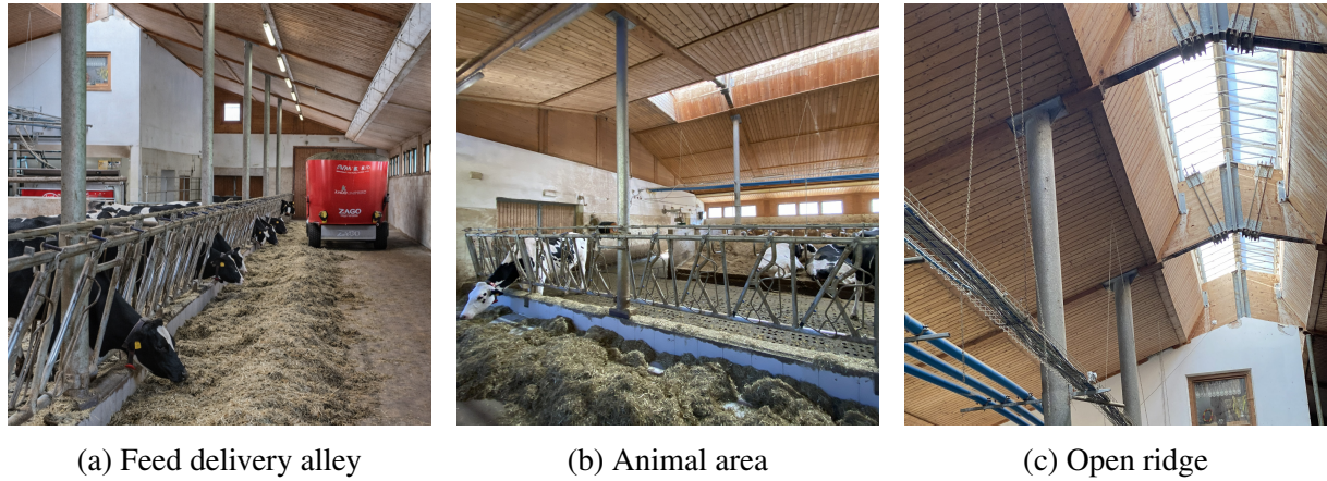
Figure 2.5: Internal areas of the cattle barn.
