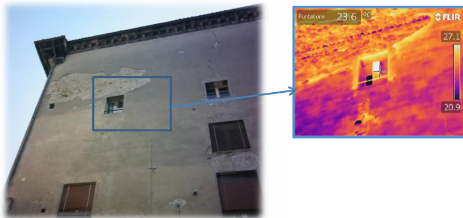
Figure 2.16: Example of thermographic measure of a facade of a building. [15]
