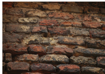
Figure 2.14: A detail of the Civic Tower in Ravenna: deposition of pollutants and black crusts are evident. [14]
