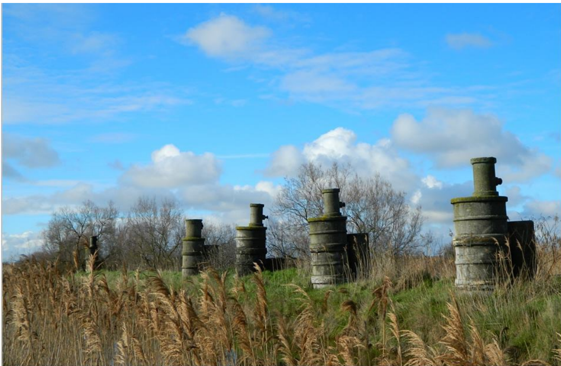
Figure 11. Compression stations in concrete
