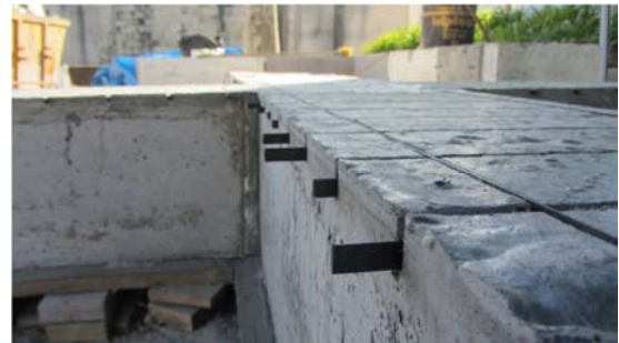
Figure 3.30 – intersection between carbon laminates
