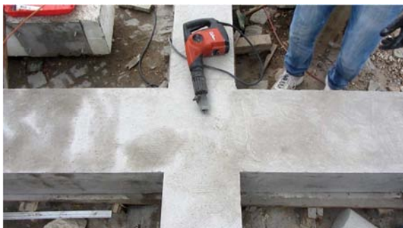
Figure 3.51 – Top surface roughened
