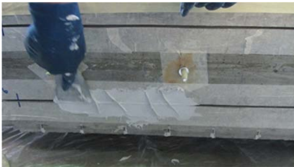
Figure 3.72 – Installation of CFRP bars into the groove.
