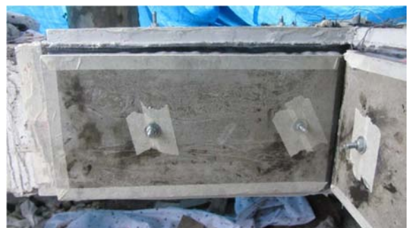
Figure 3.62 – Lateral strengthening completed
