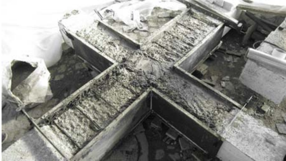
Figure 3.75 – Casting of normal concrete
