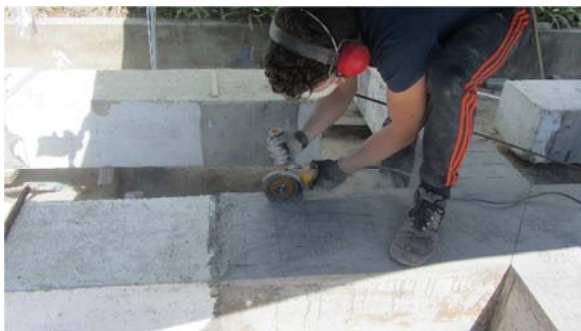
Figure 3.79 – Cutting grooves on JPA-3
