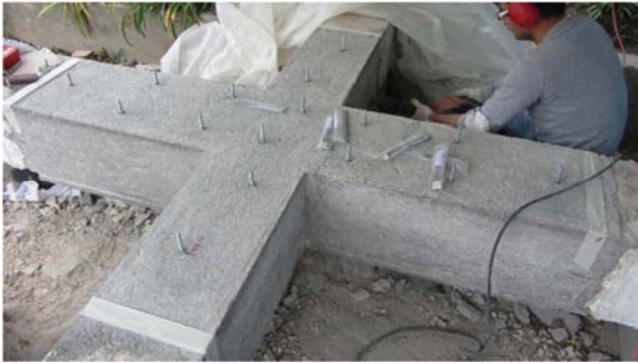
Figure 3.53 – Putting the anchors on top surface
