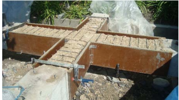
Figure 3.48 – Application of the formwork
