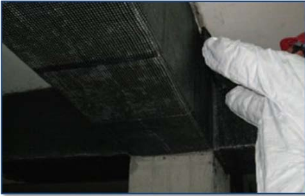
Figure 2.3 - Externally bonded FRP concrete columns [7]
