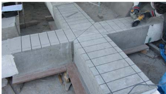
Figure 3.68 – Cutting grooves on the top surface
