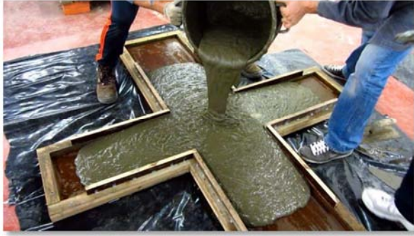
Figure 3.17 - Casting SHCC for precast panels
