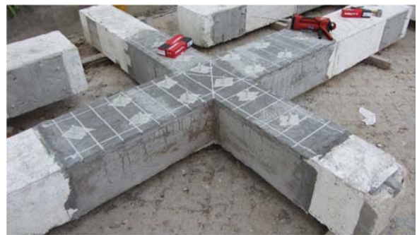
Figure 3.84 – Putting the anchors on JPA-3
