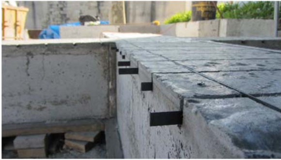
Figure 3.81 – View 1 of CFRP bars into the groove
