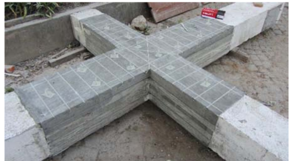
Figure 3.73 – Putting of anchors in JPB
