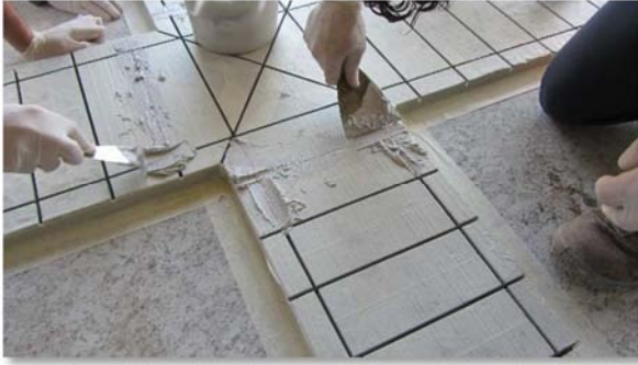
Figure 3.21 – Filling grooves with epoxy glue
