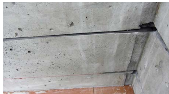
Figure 3.69 – Cutting grooves on the lateral surface
