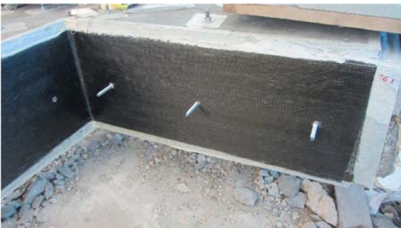
Figure 3.55 – Putting of the strain gauges
