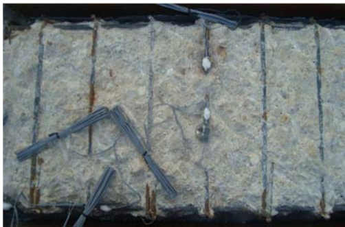
Figure 3.49 – Application of the strain gauges
