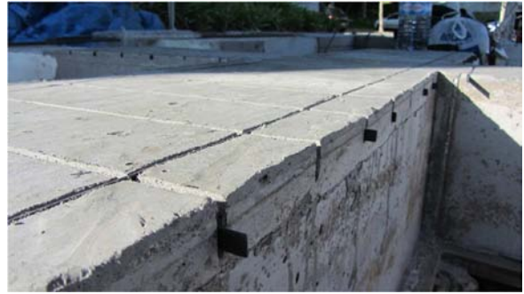
Figure 3.82 - View 2 of CFRP bars into the groove
