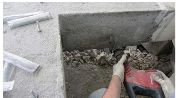
Figure 3.52 - Lateral surface roughened
