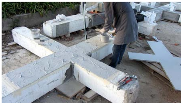
Figure 3.43 – Spreading of the glue
