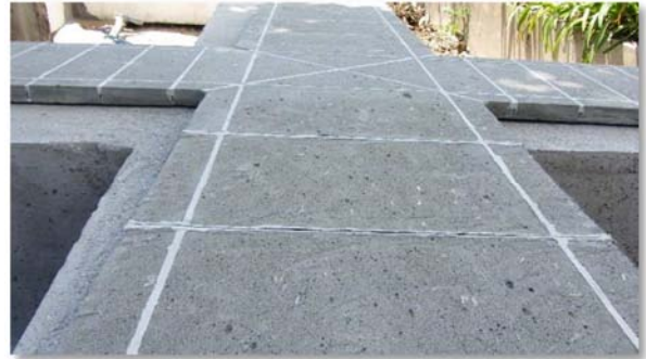
Figure 3.24 – Roughened surface ready
