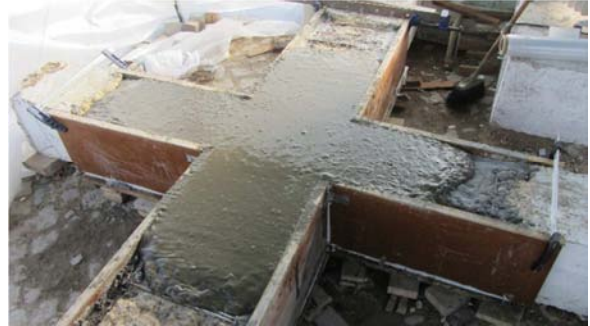
Figure 3.76 – Casting of SHCC
