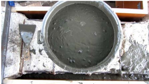
Figure 3.64 – Preparation of the mix
