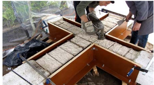
Figure 3.65 – Casting SHCC material
