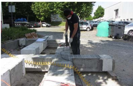
Figure 3.83 – Drilling the hole on the top surface
