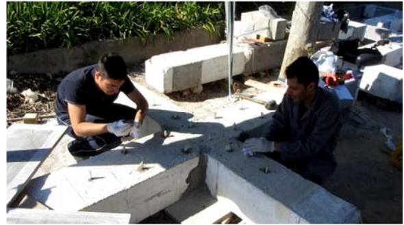
Figure 3.42 – Putting the anchors
