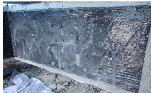
Figure 3.60 - Spreading of epoxy glue on the panel
