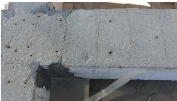
Figure 3.39 – Surface roughned
