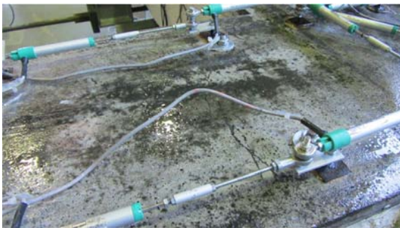
Figure 4.6 – Cracks on the beam
