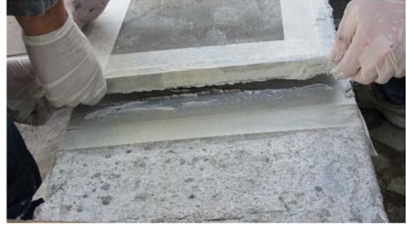
Figure 3.58 – Installation of the panel
