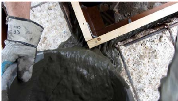
Figure 3.66- Casting SHCC material
