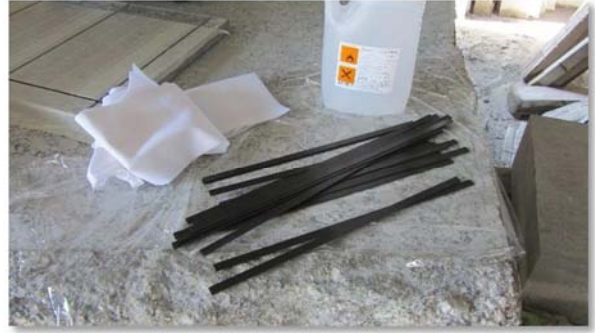
Figure 3.22 – Cleaning of carbon FRP laminates
