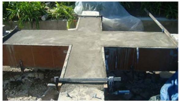
Figure 3.50 – Casting of the new concrete
