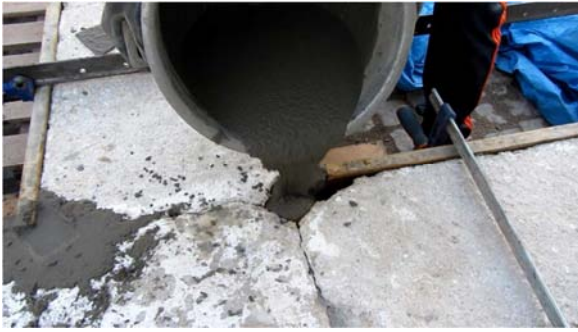
Figure 3.35 – Casting corner
