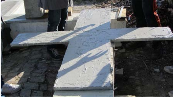
Figure 3.57 – Spreading of glue in the panel
