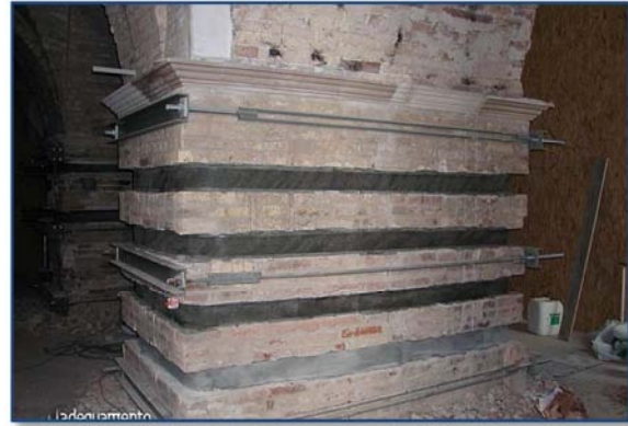
Figure 2.4 – Externally bonded FRP on masonry [7]
