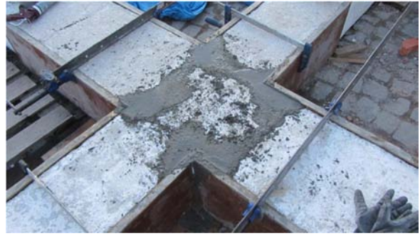
Figure 3.36 – Leveling of the surface
