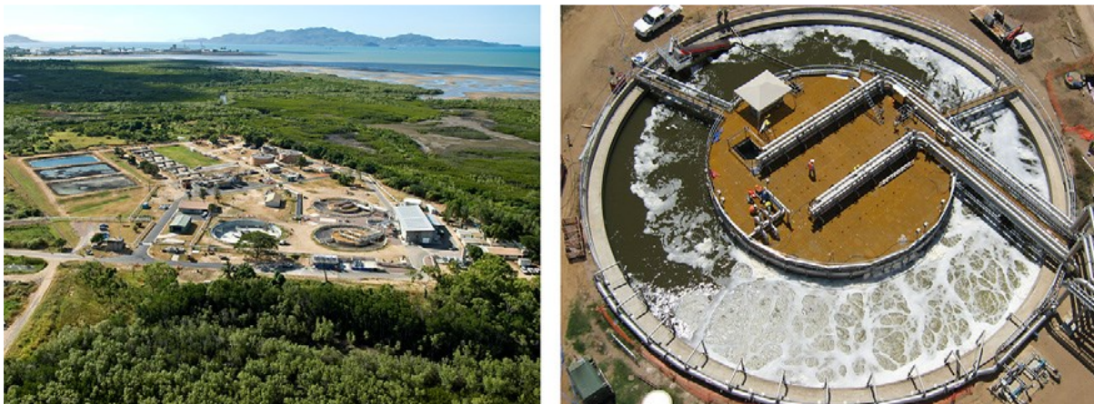
Figure 3.1: Cleveland Bay (29 MLD ADF) Wastewater Treatment Facility, Townsville. Photos taken in 2007 during MBR commissioning of (a) the site, and (b) the MBR plant, fitted into an existing old sedimentation tank. Magnetic Island (the location of Picnic Bay, the first full-scale MBR plant in Australia), is in the far distance of (a).
