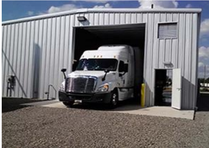
Figure 1.7. Steel workspace ( https://steelmillcranes.com/industrial-steel-structure/ )
