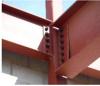
Figure 1.12. Shear connection (Brockenbrough & Merritt, 1994)
