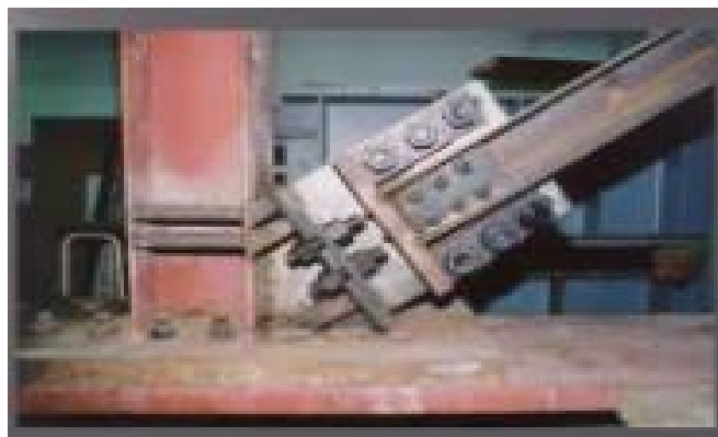
Figure 1.10. Bolted connections (Michigan et al., 2008)
