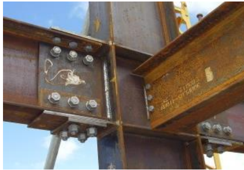
Figure 1.13. Moment connection (Brockenbrough & Merritt, 1994)
