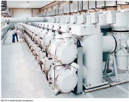
Figure 1.10: Gas-insulated Switchgear ELK-04 by ABB
