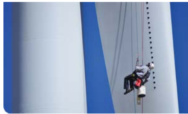
Figure 3.7: Installation of VGs on the root section of the blade [21]
